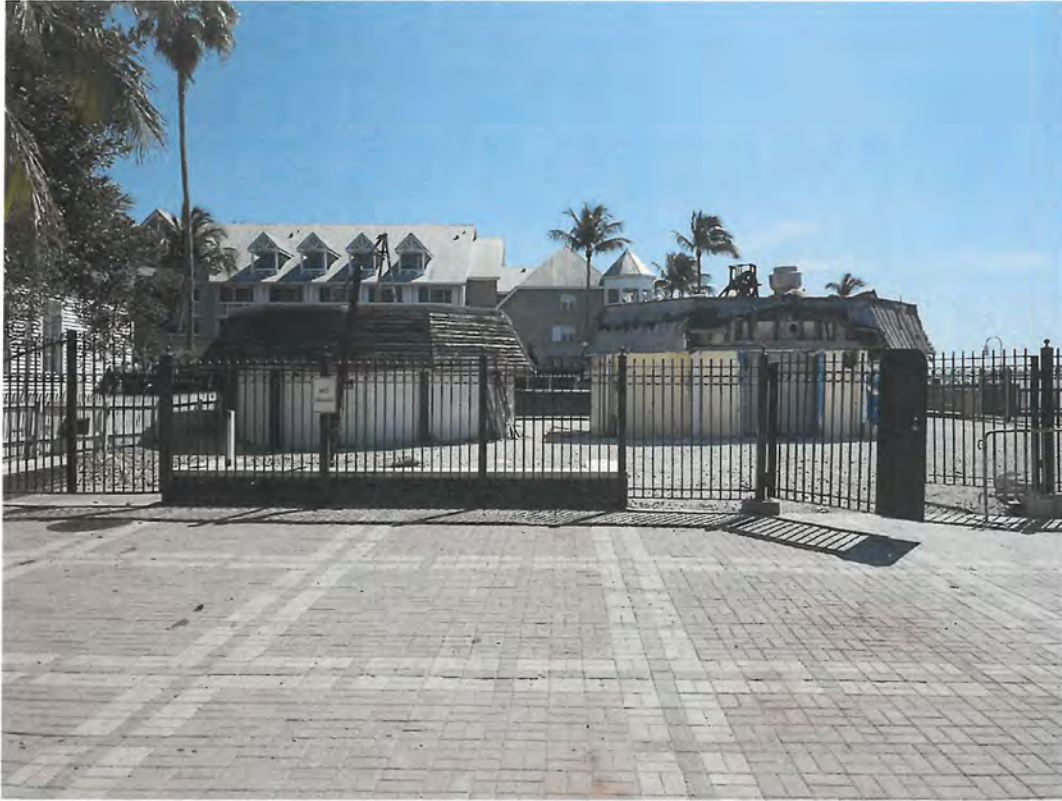
View of Cable Huts from Mallory Square. East Cable Hut is on the left, West is on the right.
