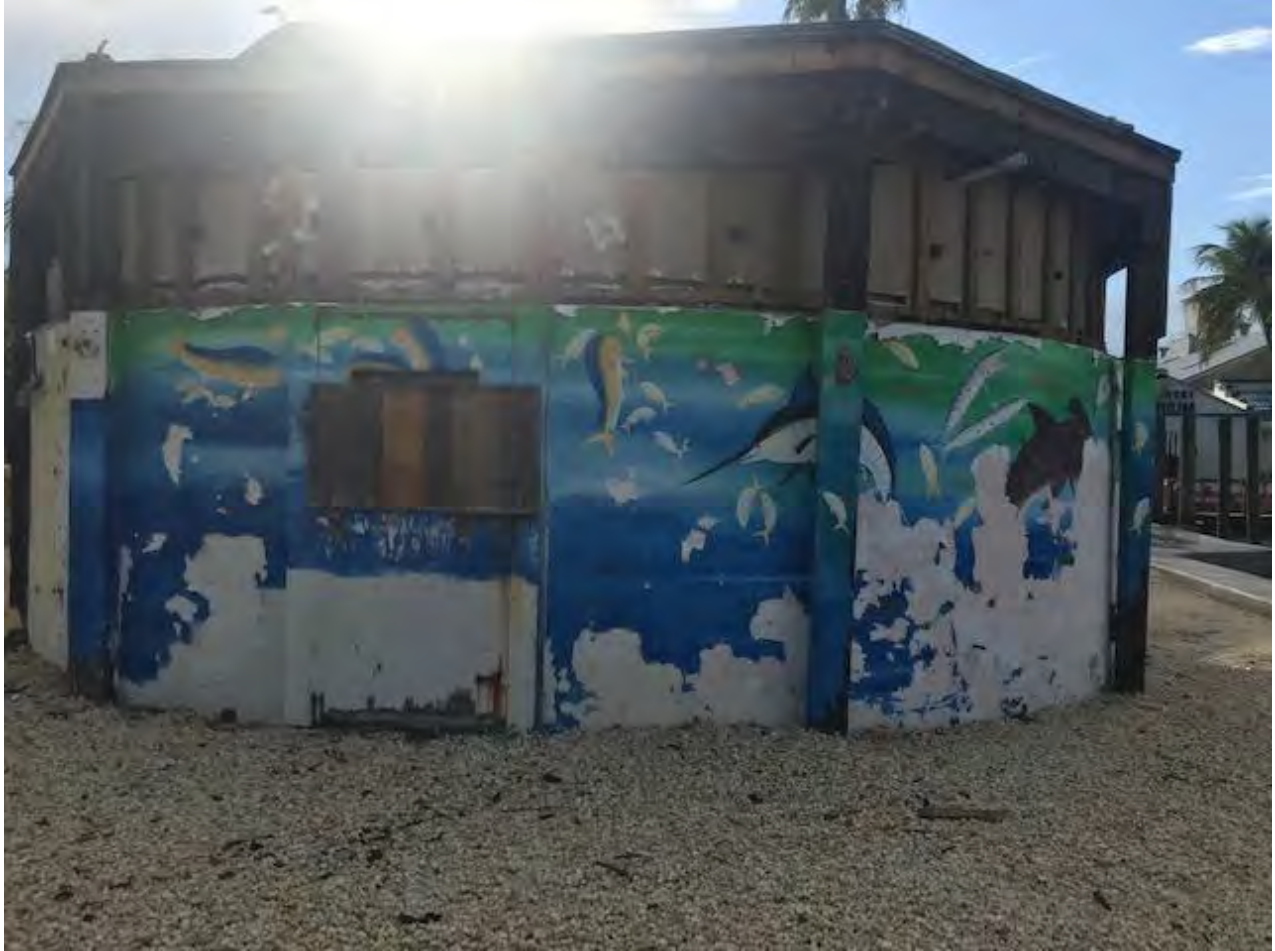
Westernmost Cable Hut photograph facing east.
