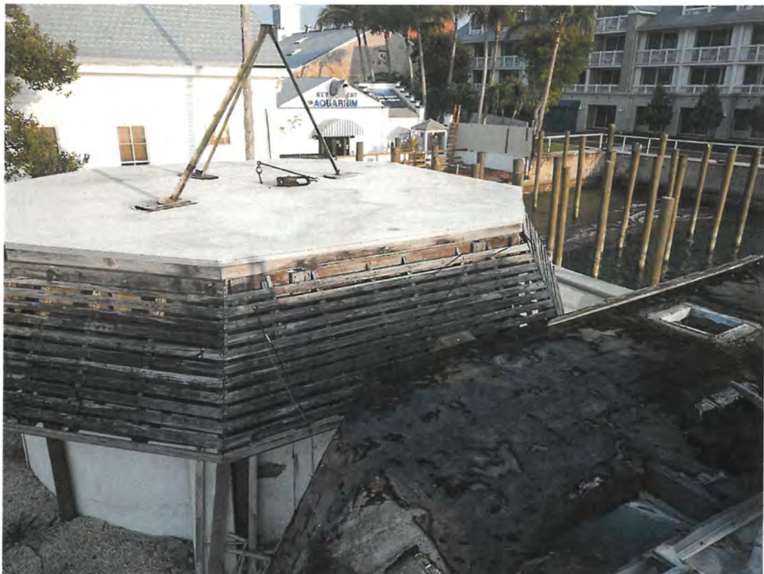
Roof of East Cable Hut.
