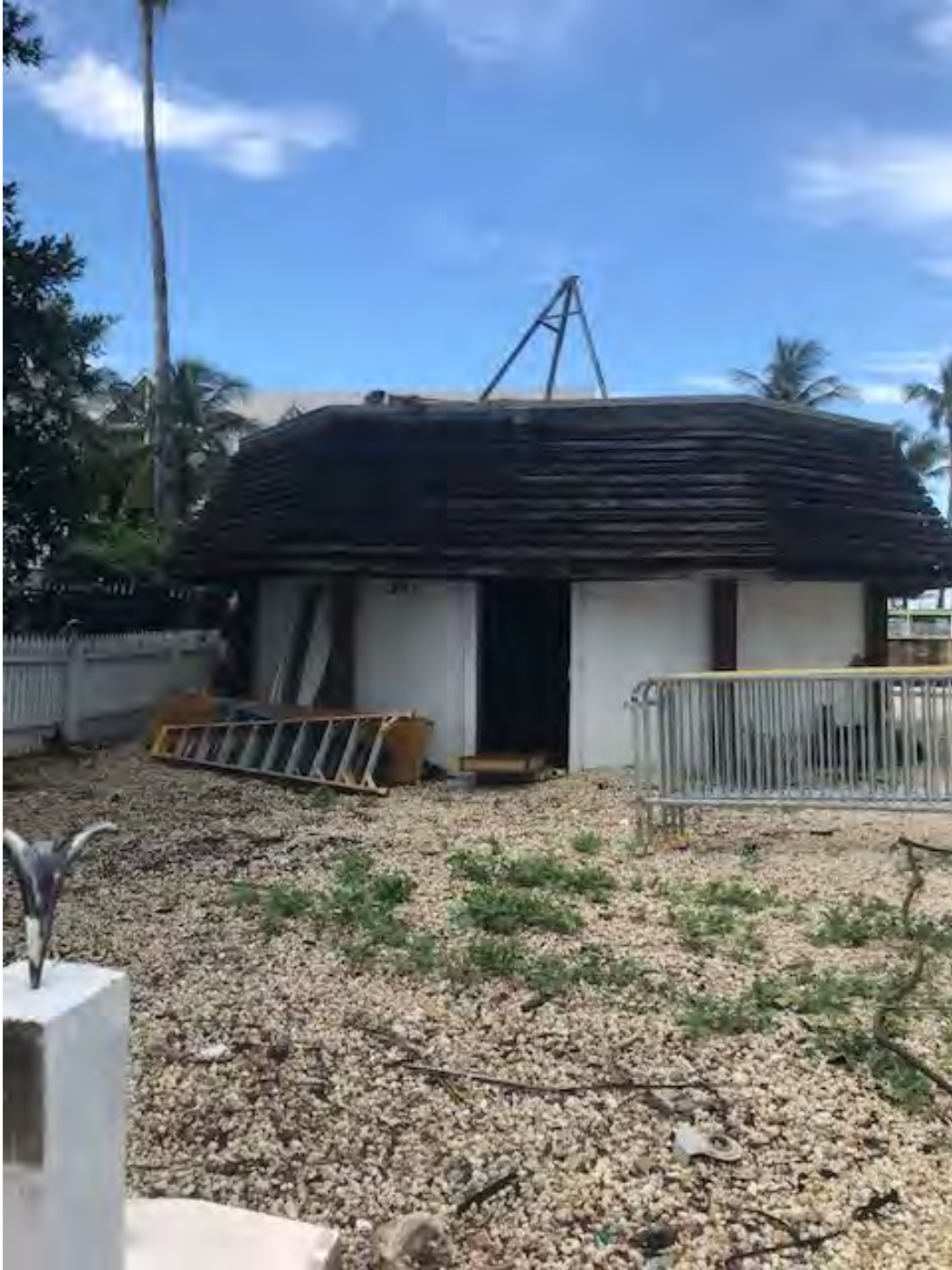
Photograph of easternmost Cable Hut from Mallory Square.
