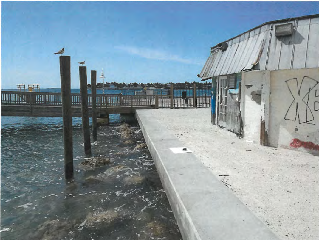
West elevation of West Cable Hut.
