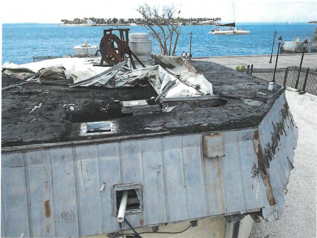
Roof of West Cable Hut.
