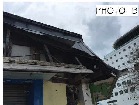
REMOVE EXISTING METAL ROOFING, ROOF FRAMING AND DETERIORATED SOFFIT
