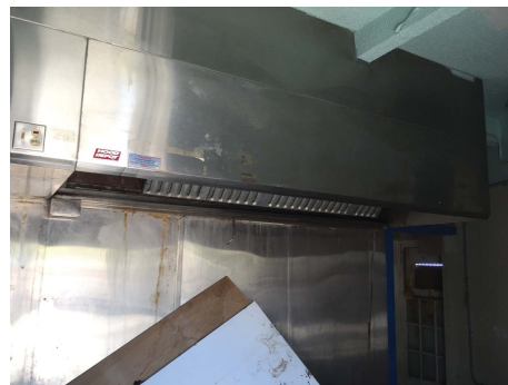
EXISTING CABLE HUT INTERIOR REMOVE ALL INTERIOR KITCHEN EQUIPMENT & NON HISTORIC MATERIALS
