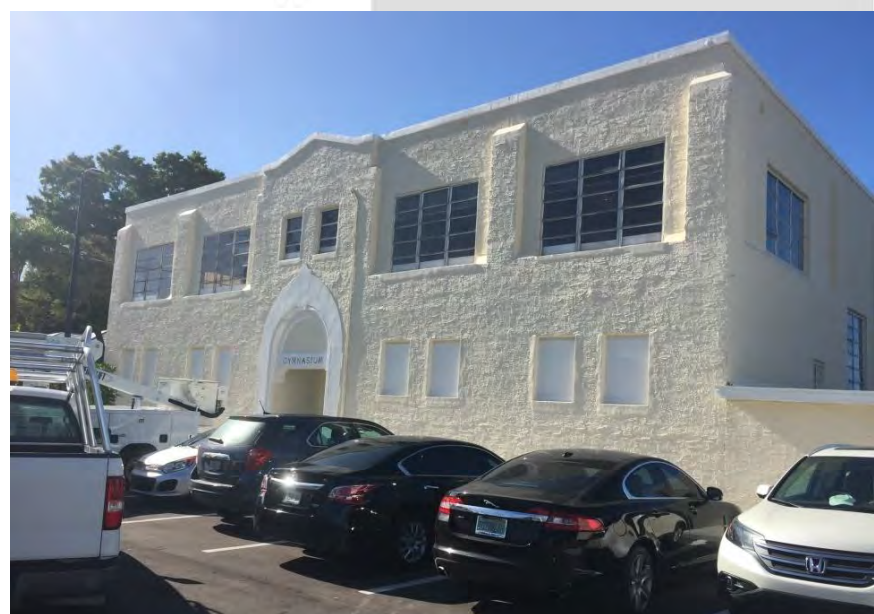
EXISTING BUILDING PRIOR TO CONSTRUCTION
