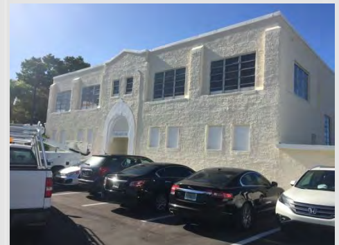
OLD GYMNASIUM BUILDING
