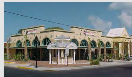
SIMONTON ROW, 120 SIMONTON ST.
