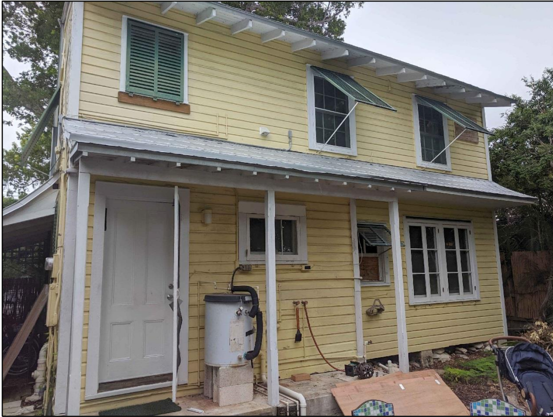
1226 South St, Existing Rear Elevation
