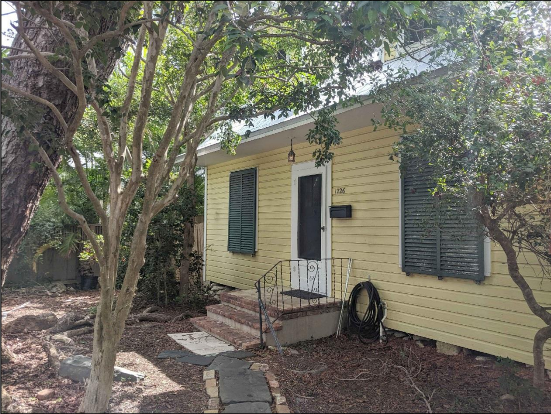
1226 South St, Existing Front Elevation.
