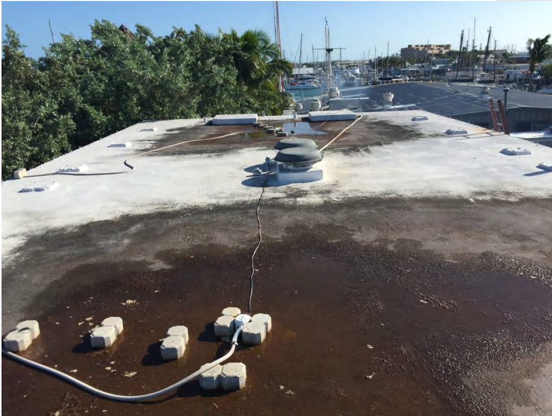
EXISTING ROOF CONDITION
