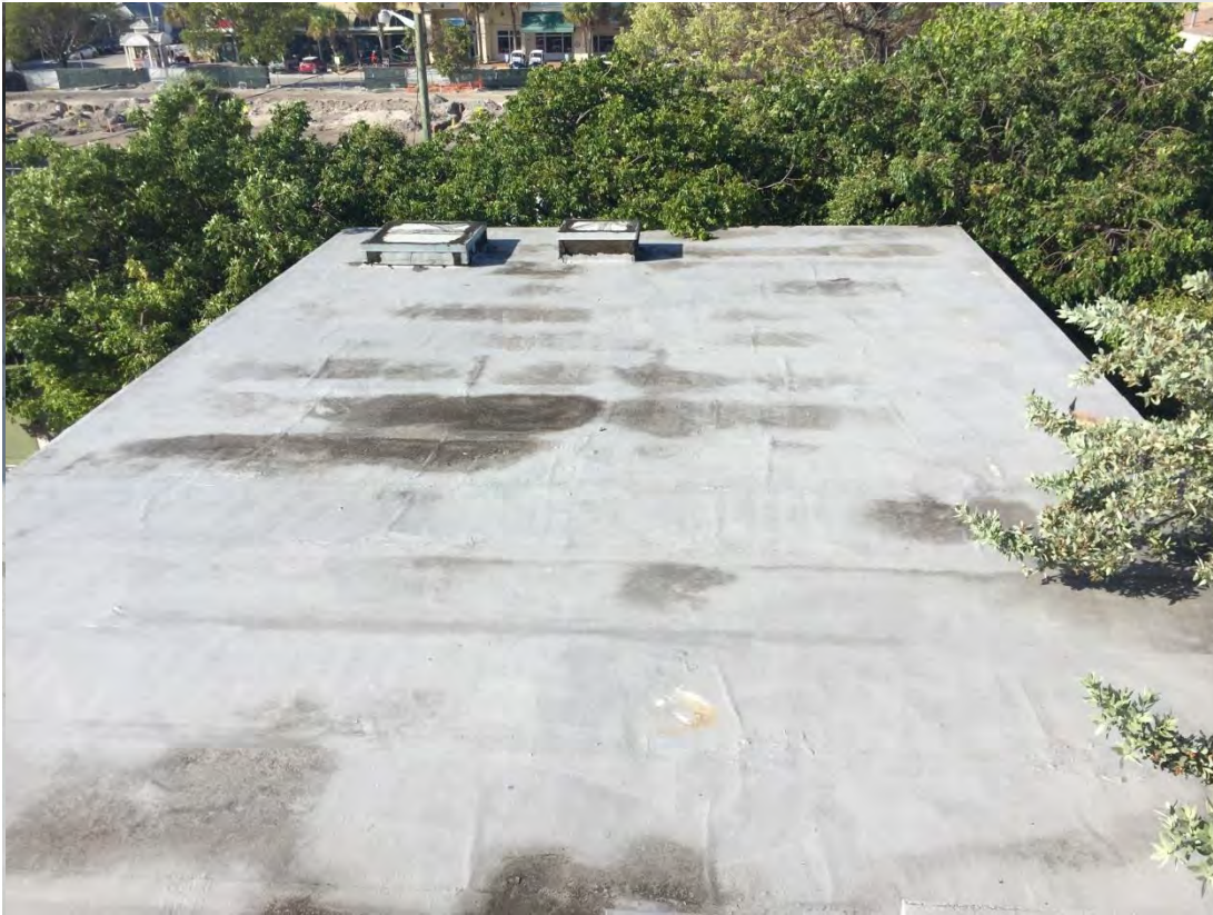
EXISTING ROOF CONDITION
