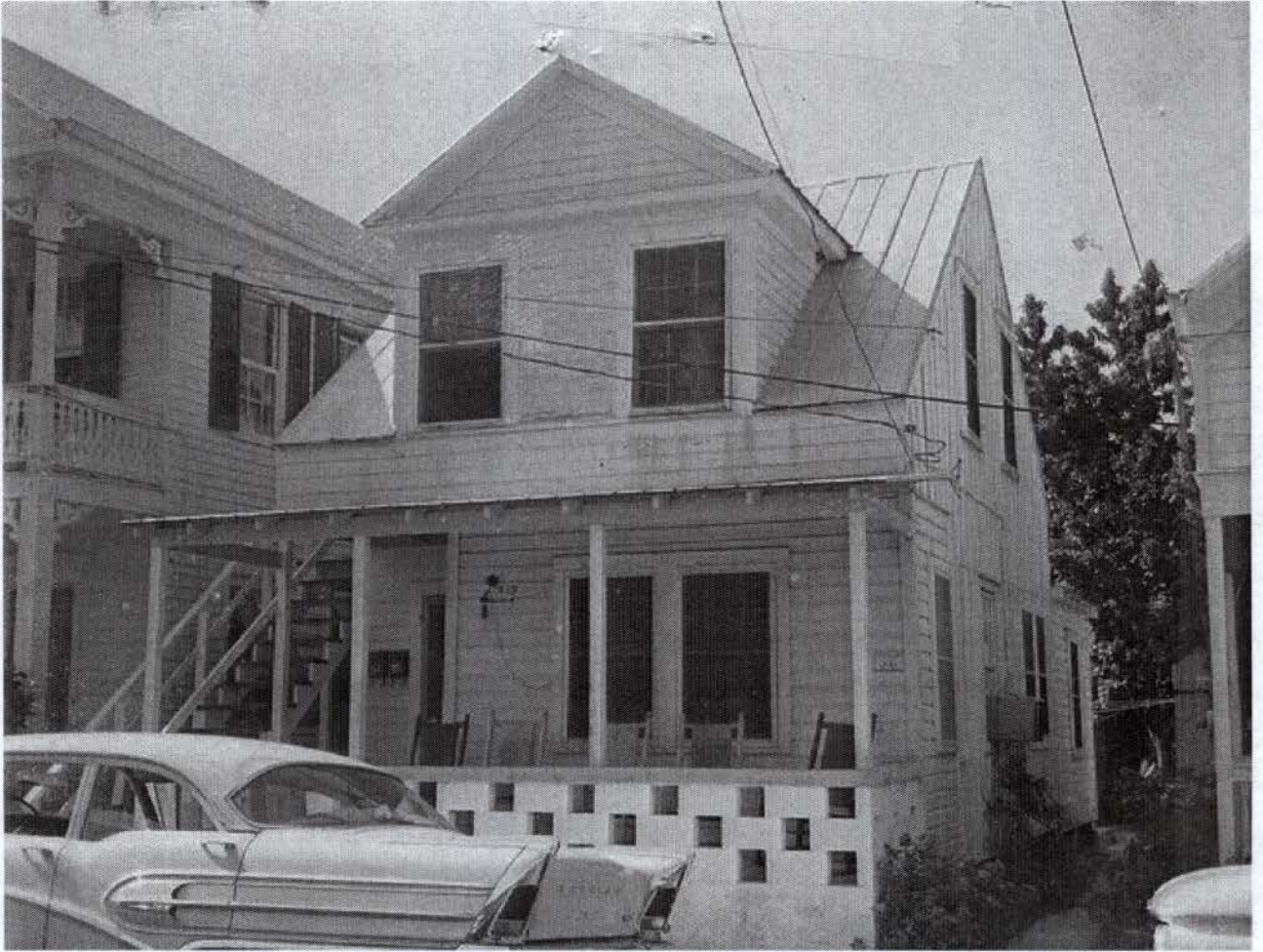
Photo taken by Property Appraiser's office c1965; 919 Southard Street; built c1889; Monroe County Library
