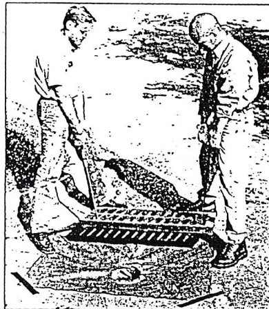
Step 2 - Insert DrainGuard. Hold in place temporarily with tape.
