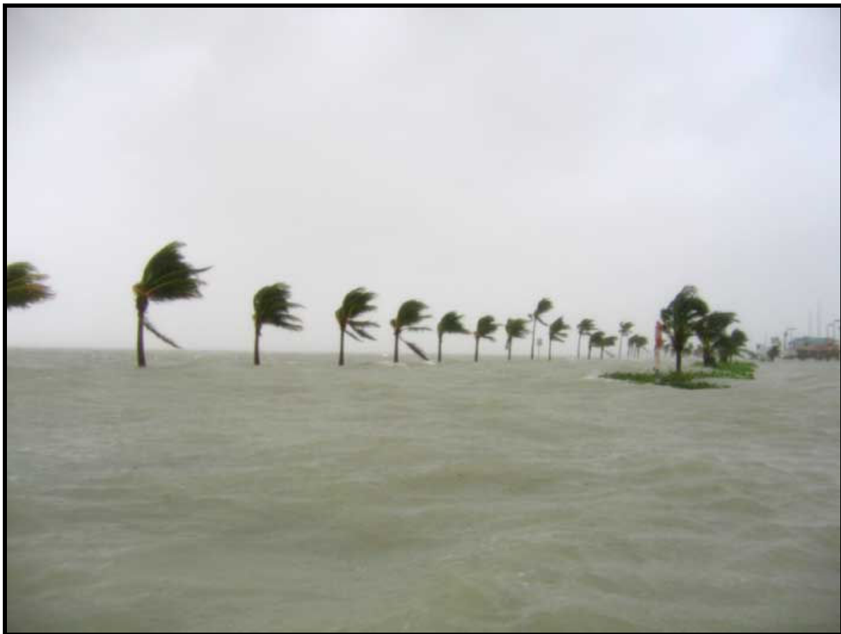
Fig. 1. North Roosevelt Boulevard, Key West, FL, inundated by a storm tide of near 6 feet (ft) above mean sea level, at approximately 0900 Eastern Daylight Time (EDT), 24 October 2005. The boulevard runs east to west, parallel to the line of coconut palm trees, on the north side of Key West (photograph by Mike Hentz of The Key West Citizen ).
