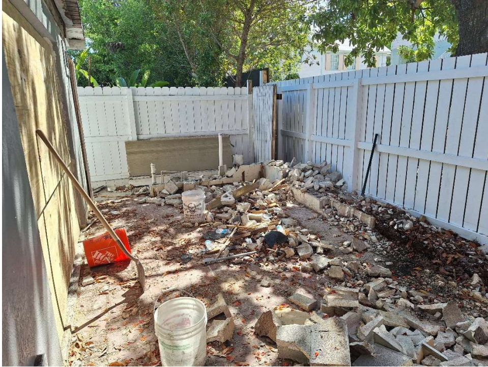
Rear yard looking west.
