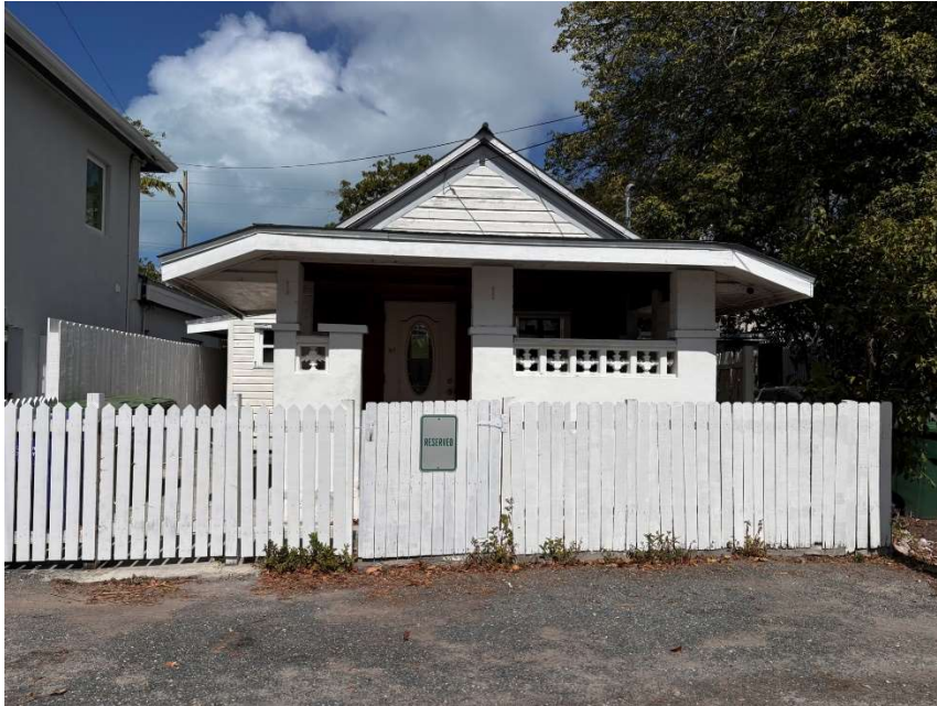
327 Julia - Front façade. Large front porch overhang to be removed and front porch to be restored to 1892 configuration.
