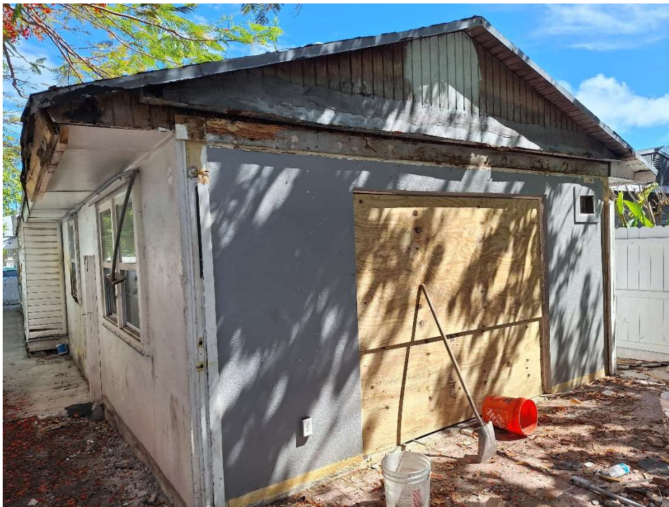
Rear (North) façade. Rear of building is CBS construction.
