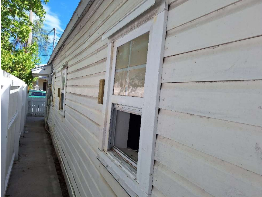
Side (East) Elevation. Front of building is wood framed. All existing windows are contemporary.
