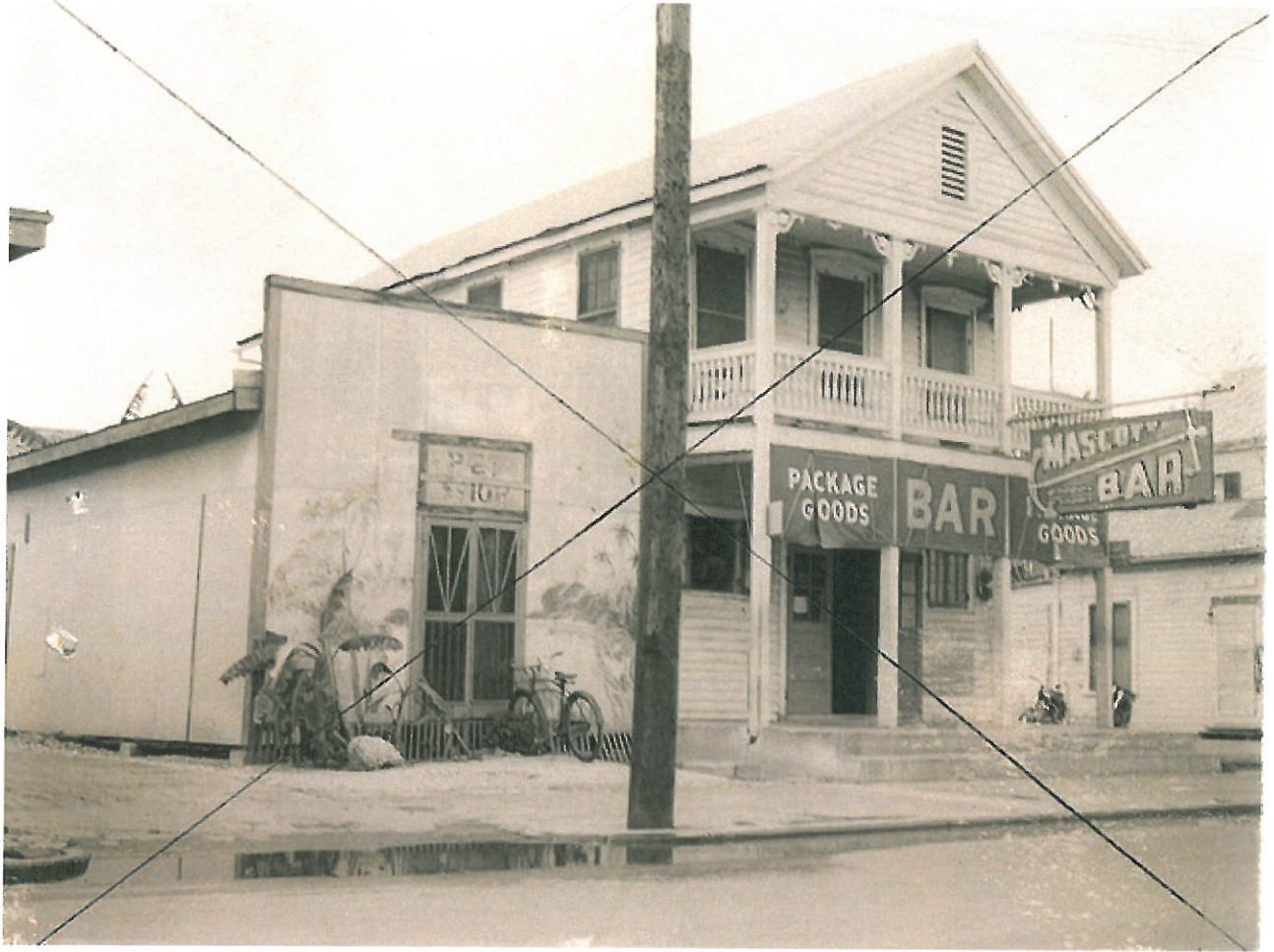
Photo taken by Property Appraiser's office c1965; 812 Caroline Street; Mascot Bar; razed abt 1970; Monroe County Library
