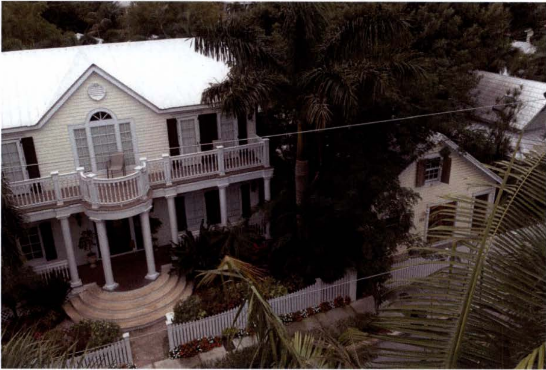
FRONT ELEVATION & NEIGHBORING STRUCTURE
