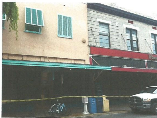
Duval Street – turnbuckle support above
