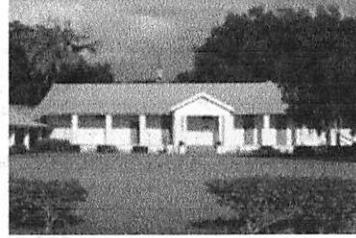
Glover School (Plant City, FL)
