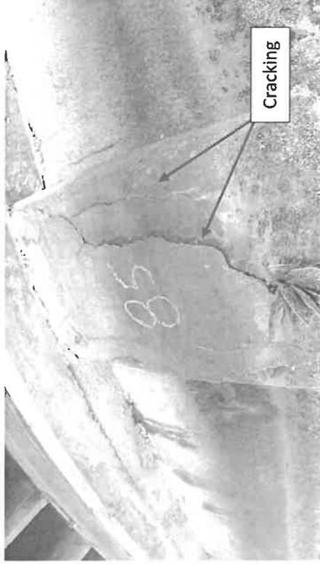
Deficiency B-86: Pile 127 (Station 9+31)
