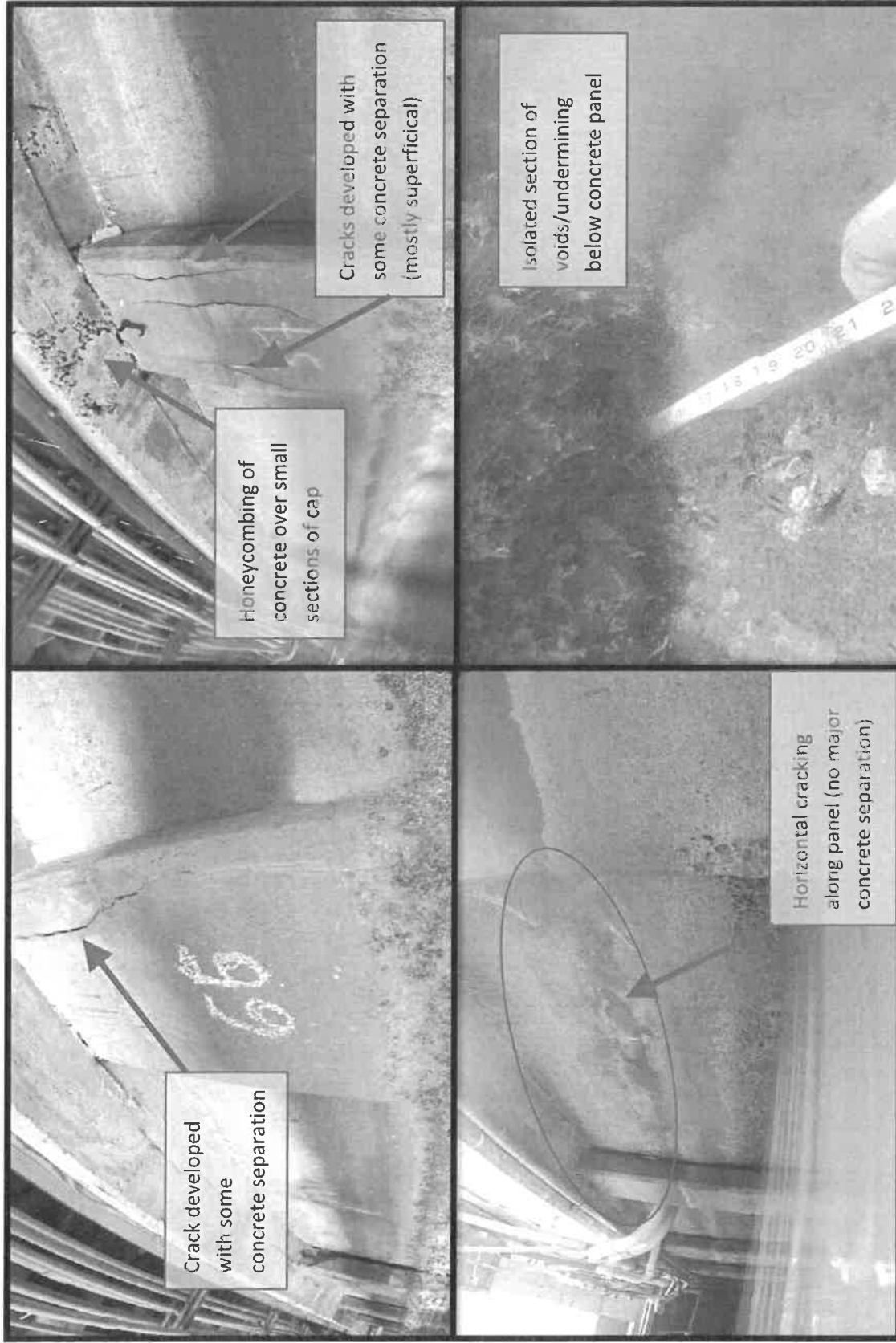
Figure 8: Typical Moderate Deficiencies – [Top Left] B-70 (Station 7+86), [Top Right] B-53 (Station 5+48), [Bottom Left] B-26 (Station 2+86), [Bottom Right] B-102 (Station 10+06)
