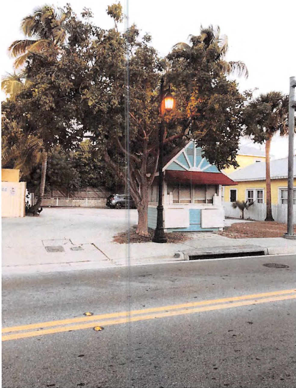
View of 511 Truman Avenue site fronting Truman Avenue. Small ticket booth/kiosk in site foreground.
