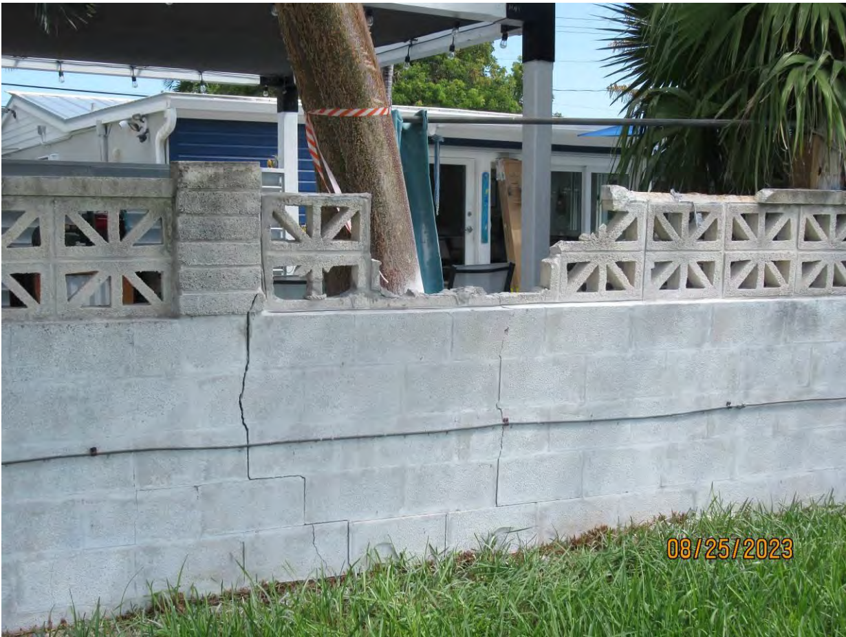
Photo showing tree trunk and property line wall damage, view 1.
