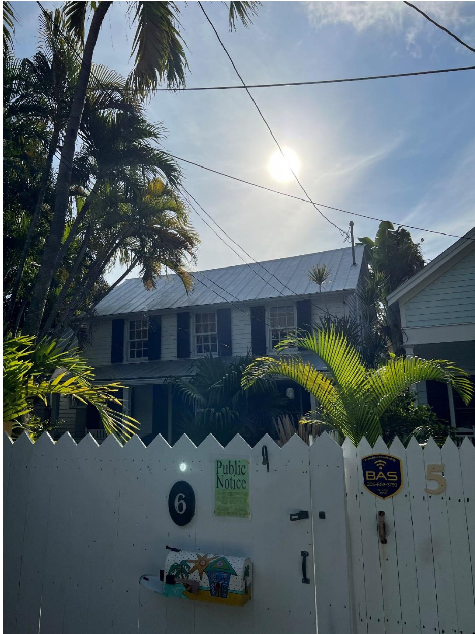
View from fence at Fletcher Ln.
