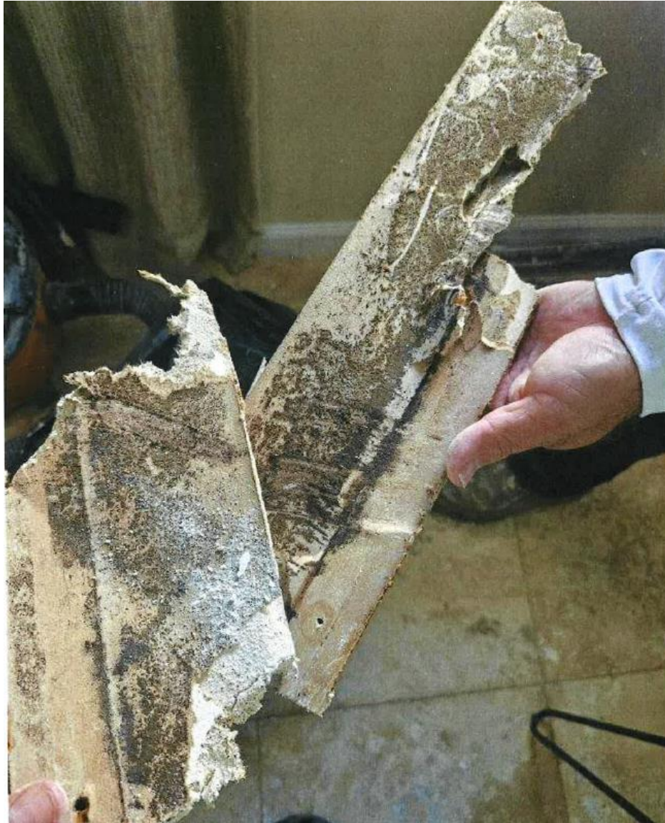
Photo of black mold found on accessory structure.
