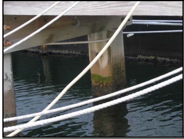
Wood deck and framing on concrete piles.
