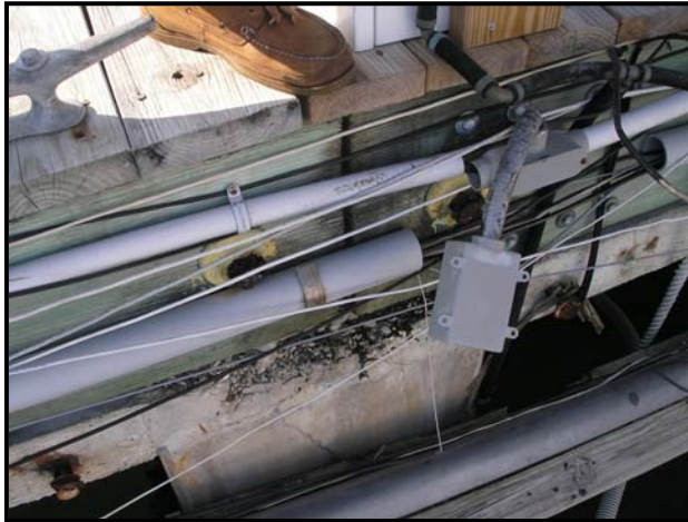
Photo of wood deck and wood substructure resting on concrete deck supported by concrete pilings encased on a concrete cap.
