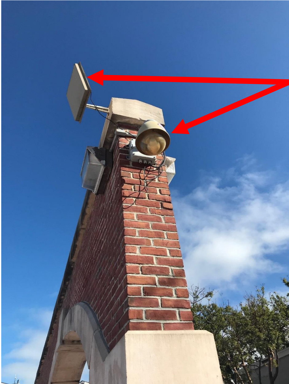
Old cameras/antennas on arches at Mallory
