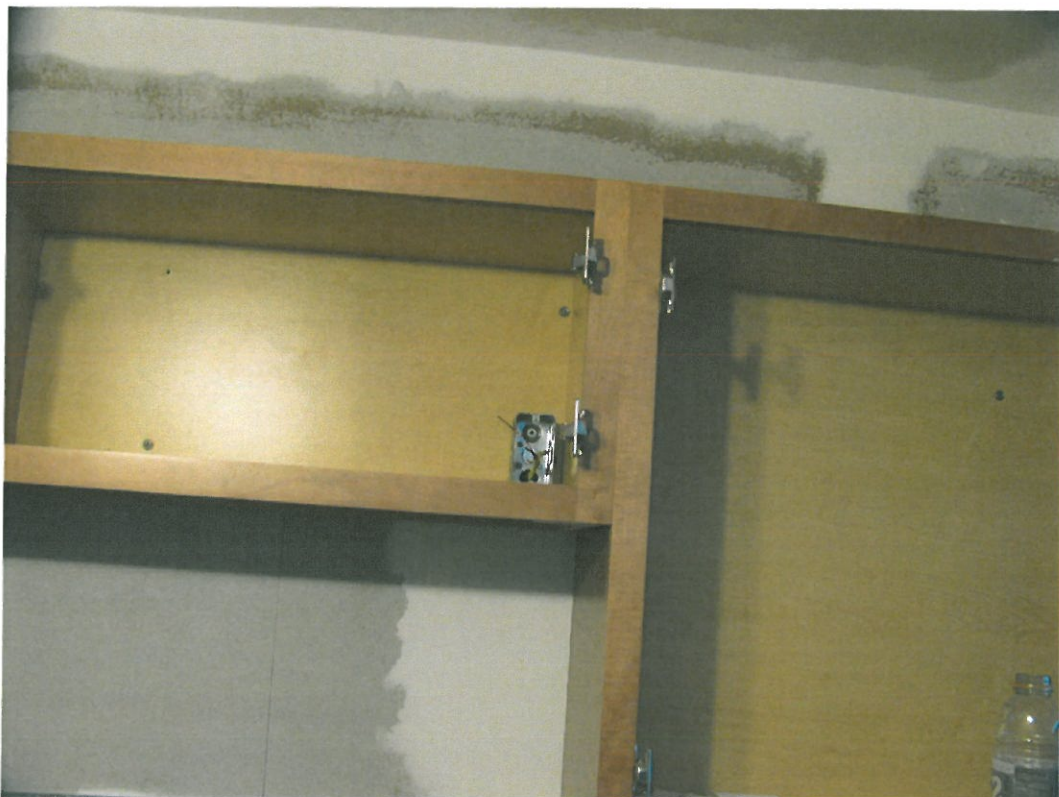
Work being performed by Mr. Roloff on 2 October 2013 Photo taken by Inspector D Ray. Cabinet backing installed to a newly installed drywall with wet paste.
