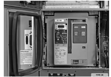
Bellows and Two-Point Door Latch
