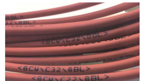
Control Wire Marking
