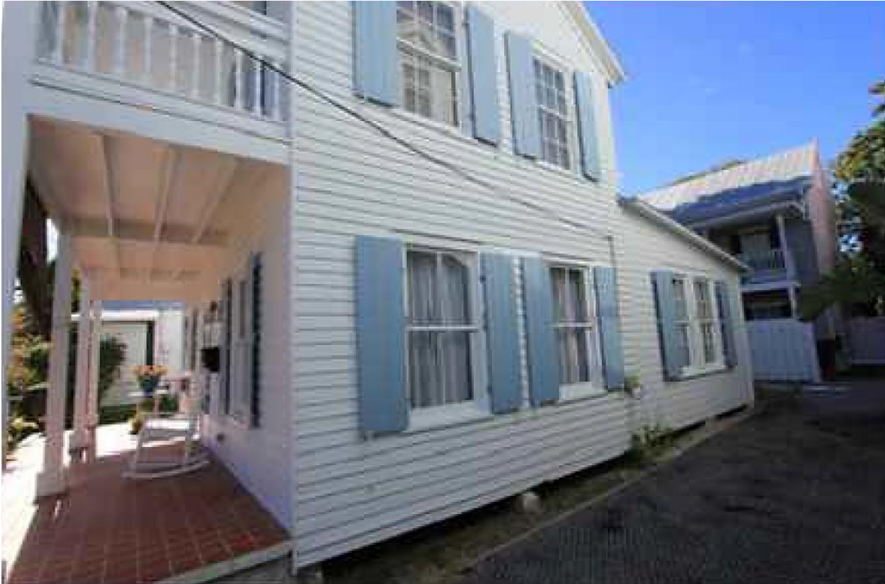
View Looking Toward Back of House
