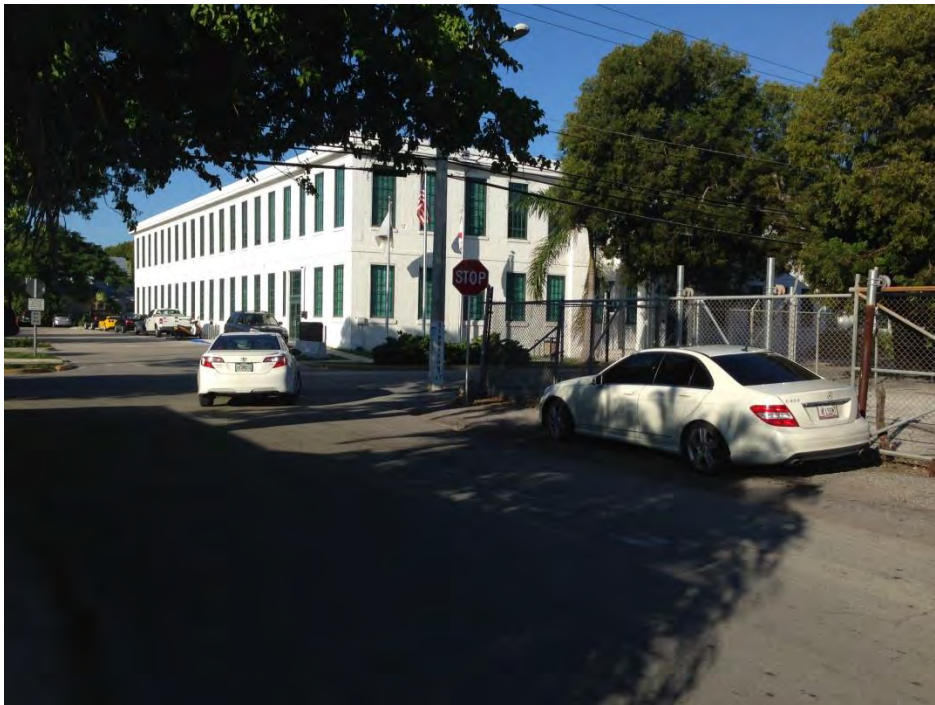
6. Photograph of the Gato Building on Simonton Street. The commercial property across Amelia Street is shown in the background.
