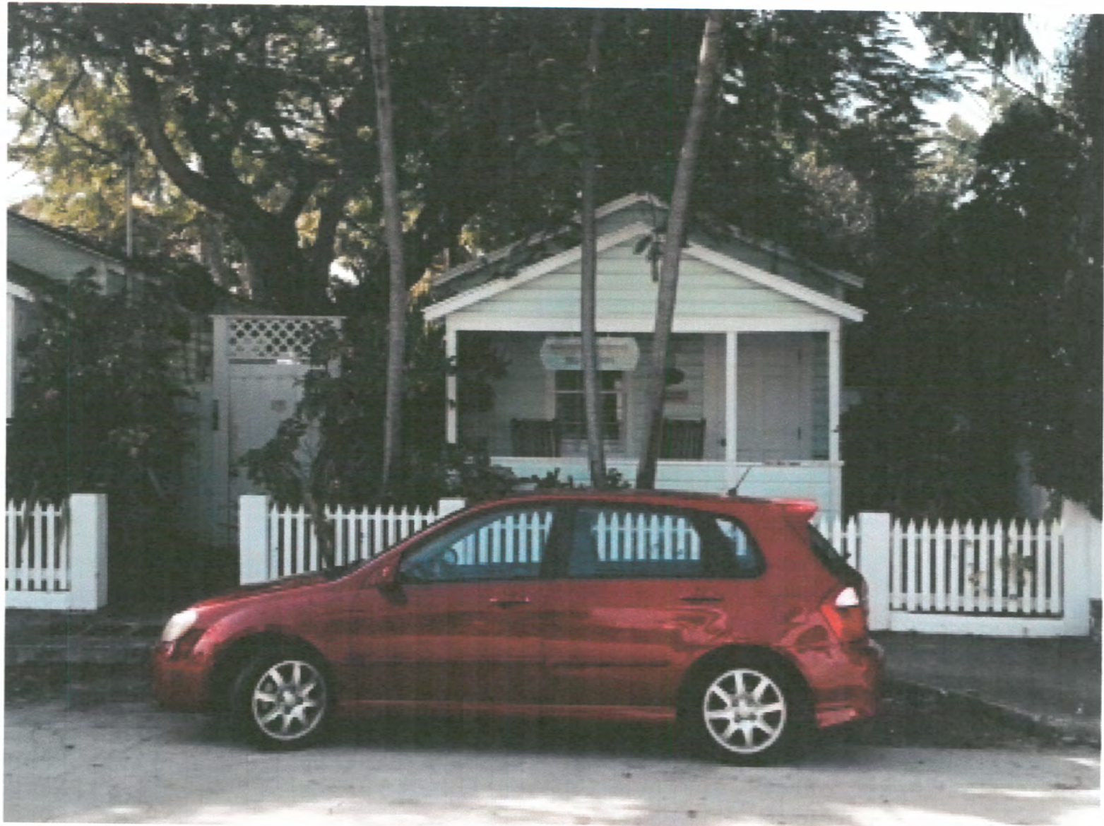
ADJACENT PROPERTIES – 1124 MARGARET ST. (ACROSS THE STREET)
