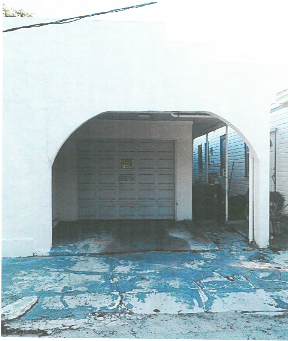
EXISTING CONDITIONS – 1111 MARGARET ST. (PORTICO FROM FRONT)
