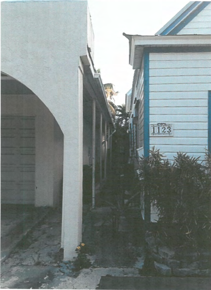
EXISTING CONDITIONS – 1111 MARGARET ST. (SOUTH SIDE VIEW)
