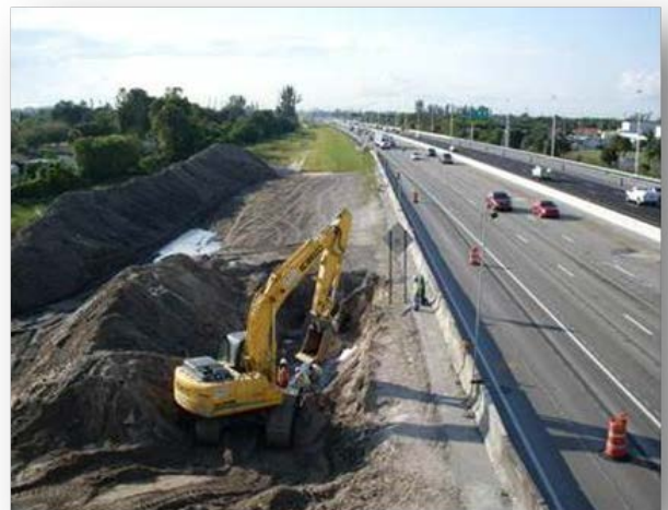
HCR working on ACM
