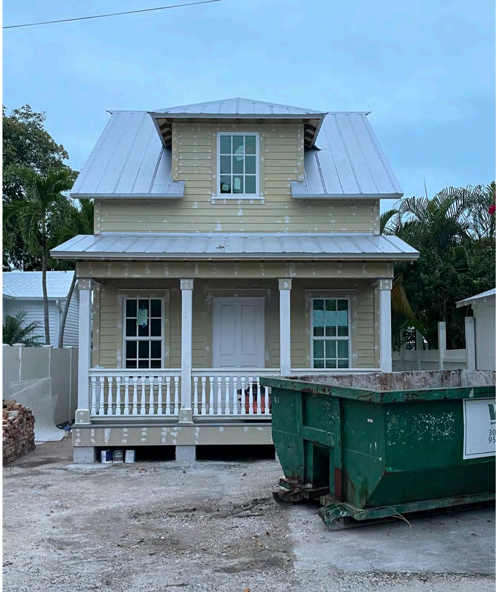
1324 DUNCAN STREET - NORTH WEST ELEVATION
