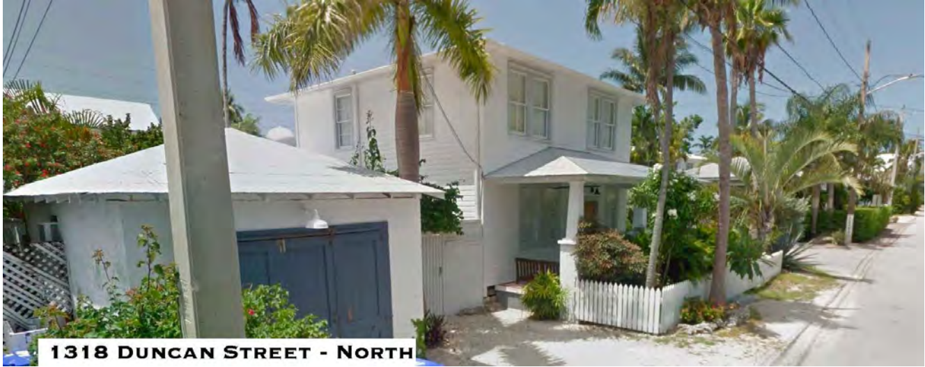
1318 Duncan Street – adjacent to subject site (southeast corner).
