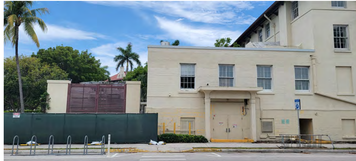
VIEW OF CHILLER FROM SEMINOLE
