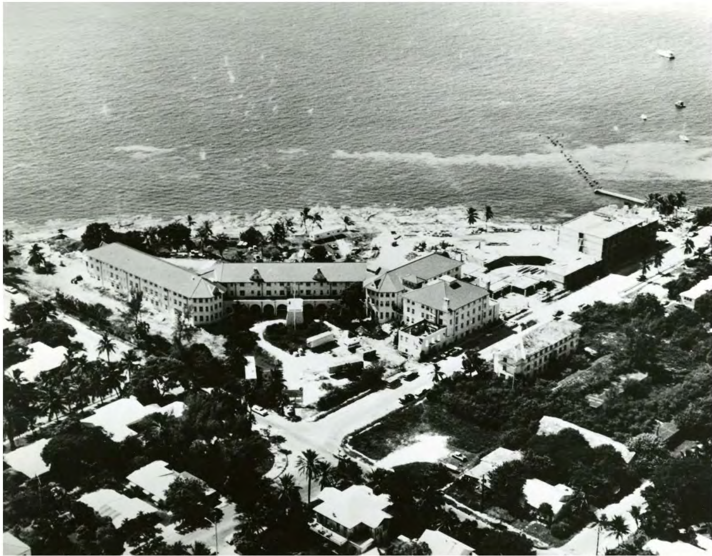
Aerial photograph of Casa Marina circa 1978. Monroe County Library.
