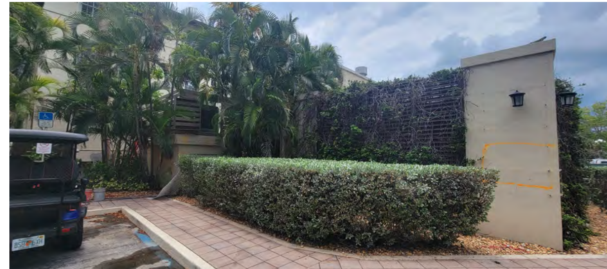
VIEW OF CHILLER FROM PARKING
