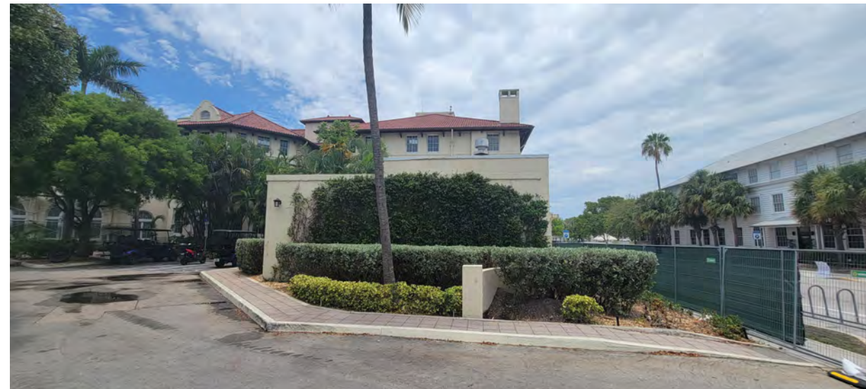
VIEW OF CHILLER FROM DRIVE
