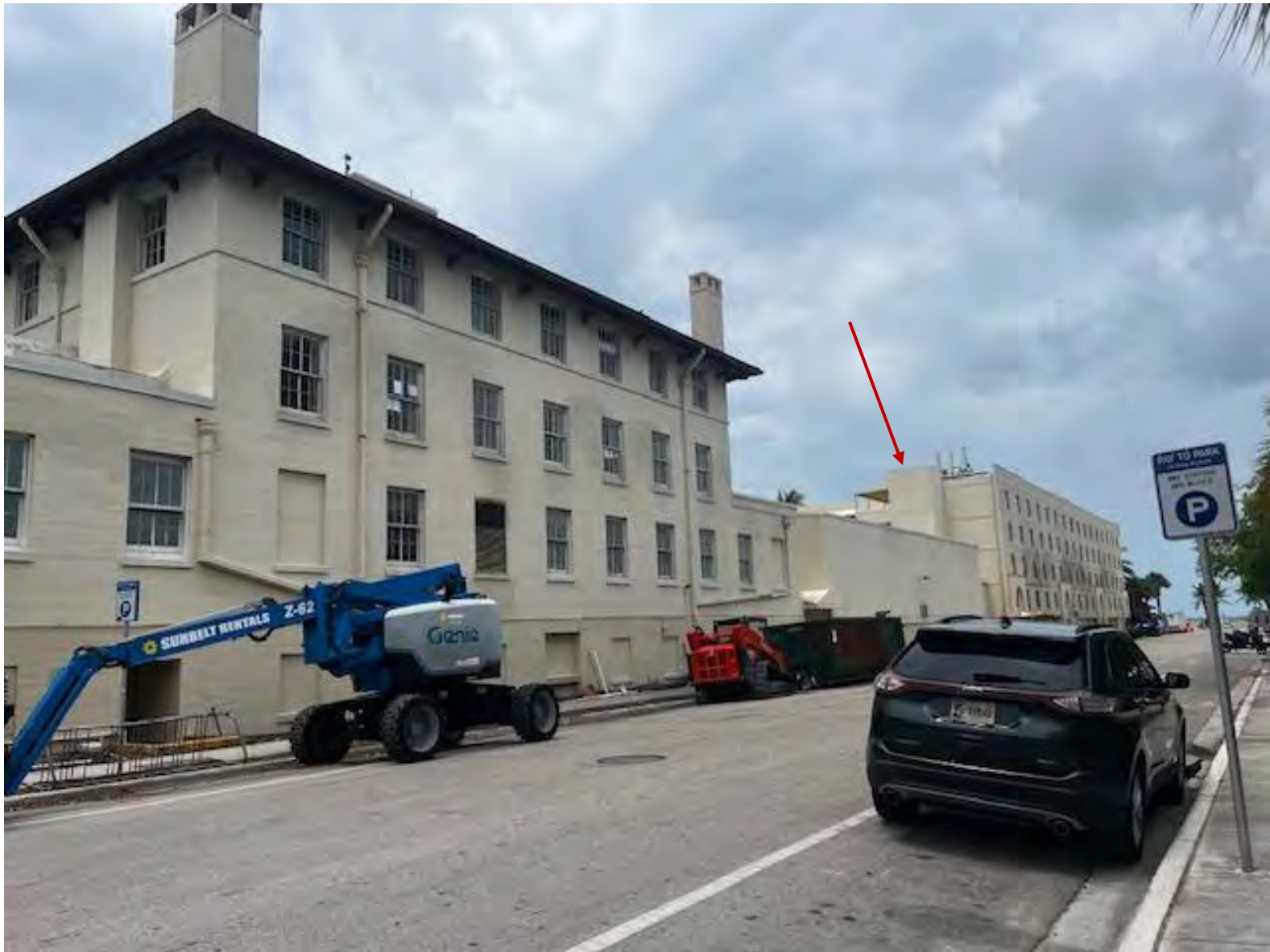
View of north elevation. Historic part of the hotel towards the left.
