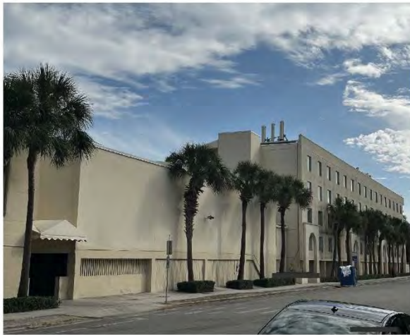
CURRENT ELEVATOR TOWER View from Seminole St.
