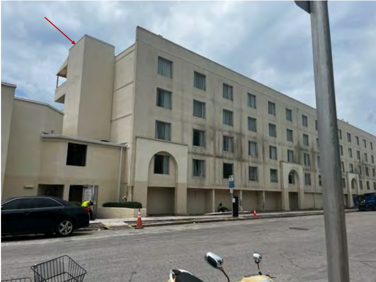
Closer look at addition with existing elevator shaft facing Seminole Avenue.
