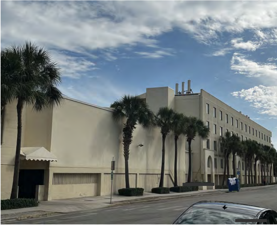
CURRENT ELEVATOR TOWER View from Seminole St.
