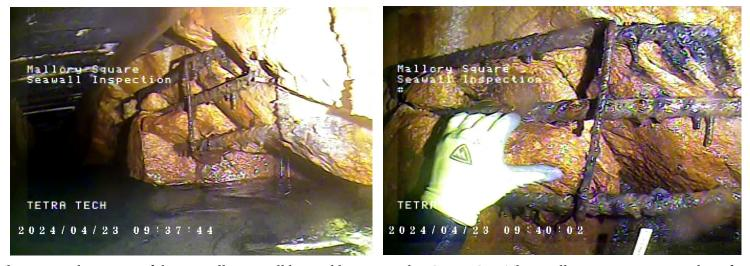
The next 2 photos are of the seawall cap spall located between piles C15 & C16. This spall area is approximately 10ft long x 24" high (full front face of Cap) x 7" to 23" deep (to sheet pile). There are 3 horizontal 1" diameter rebars (north-south), 2 horizontal 1" diameter rebars (east-west), and 2 vertical 1/4" diameter rebars exposed at this location. The expose rebars have surface corrosion and minor section loss (5%).
