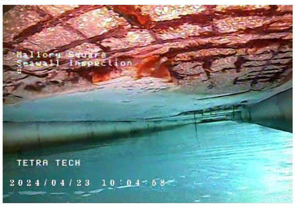
Photo is of the exposed rebar grid with rebar hanging down on the ceiling panels between the support Bents B (middle north-south support bent) & C (eastern north-south support bent by seawall) in the general area between piles 24 to 26 (looking southeast). The exposed grid spans the entire east/west distance between Bent B & Bent C and spans approximately 12' in the north/south direction. The diver counted 6 pieces of rebar hanging down.
