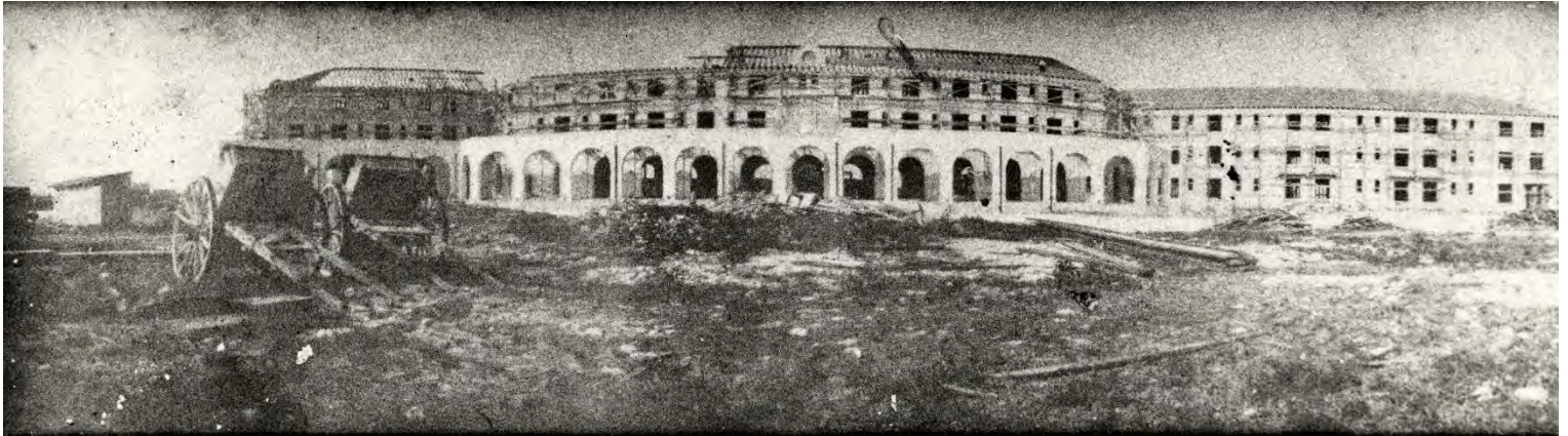
Casa Marina Resort under construction 1920. Monroe County Library
