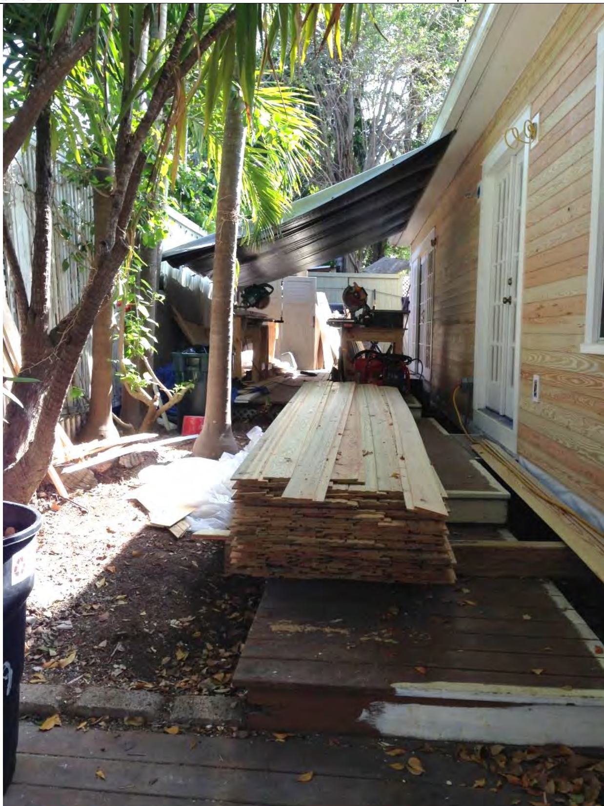
2. 1019 Varela Street- Left Side View
