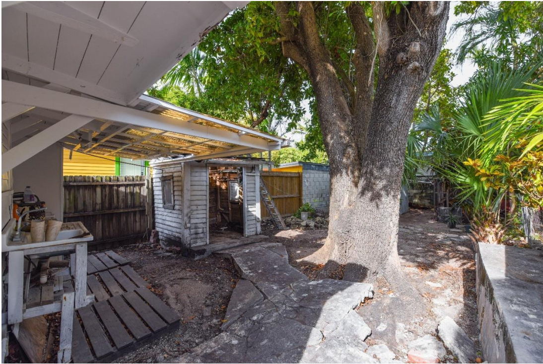
Rear non-historic additions and structures
