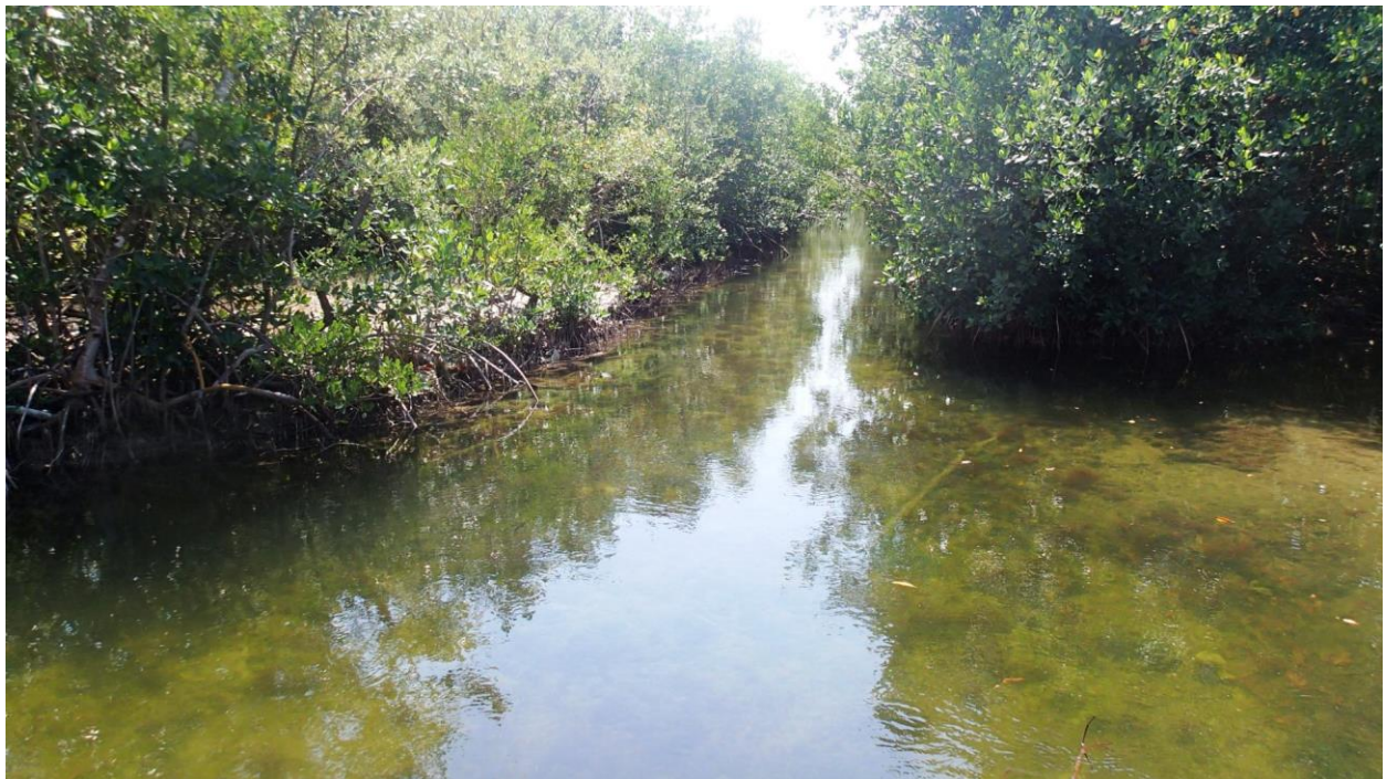
Photo of the Venetian Drive channel looking south and showing mangrove branches and roots encroaching into the conveyance.
