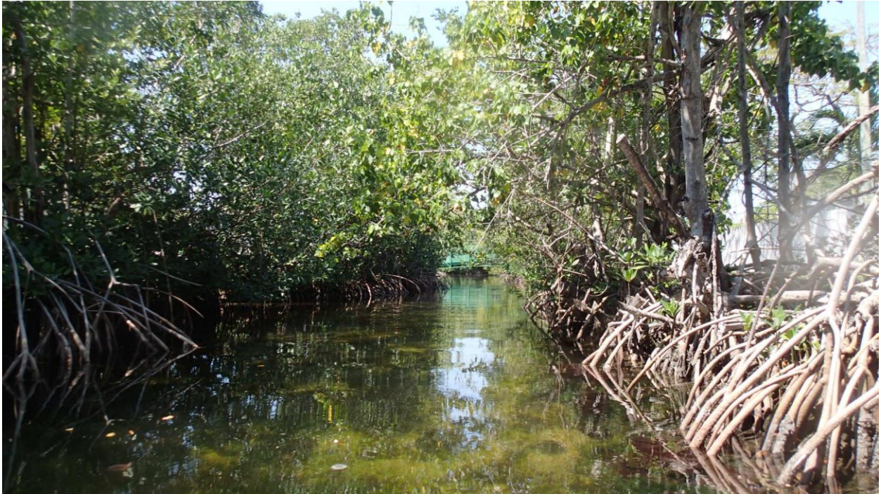
Photo of the Riviera Canal showing mangrove branches and roots encroaching into the conveyance.
