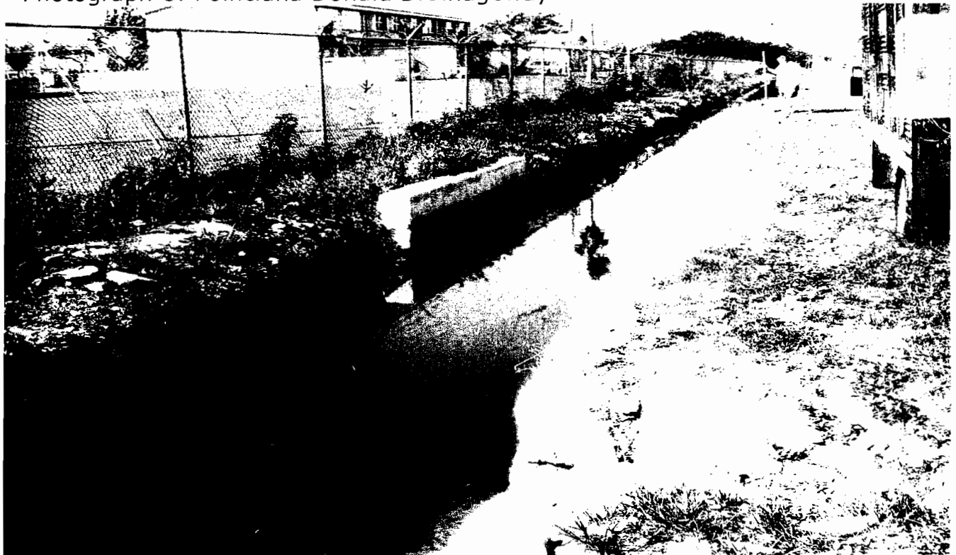
Photograph 7: Poinciana Donald Drainageway
