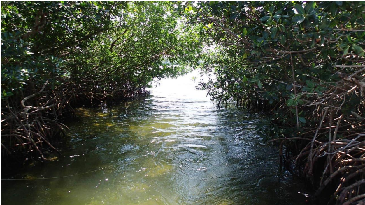
Photo of Government Road looking south from culvert showing mangrove branches and roots encroaching into the conveyance.
