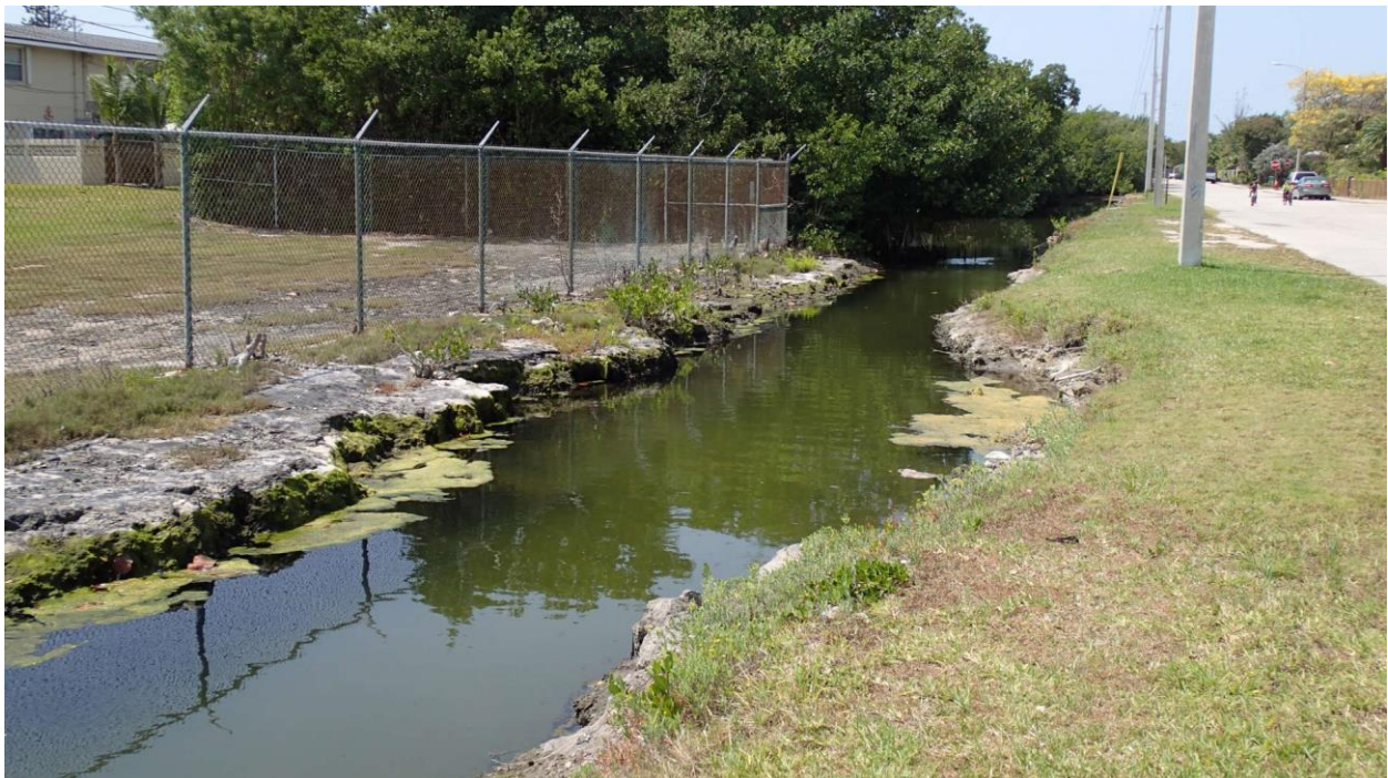
Photo of Donald Avenue channel showing accumulation of algae growth and debris in the system.
