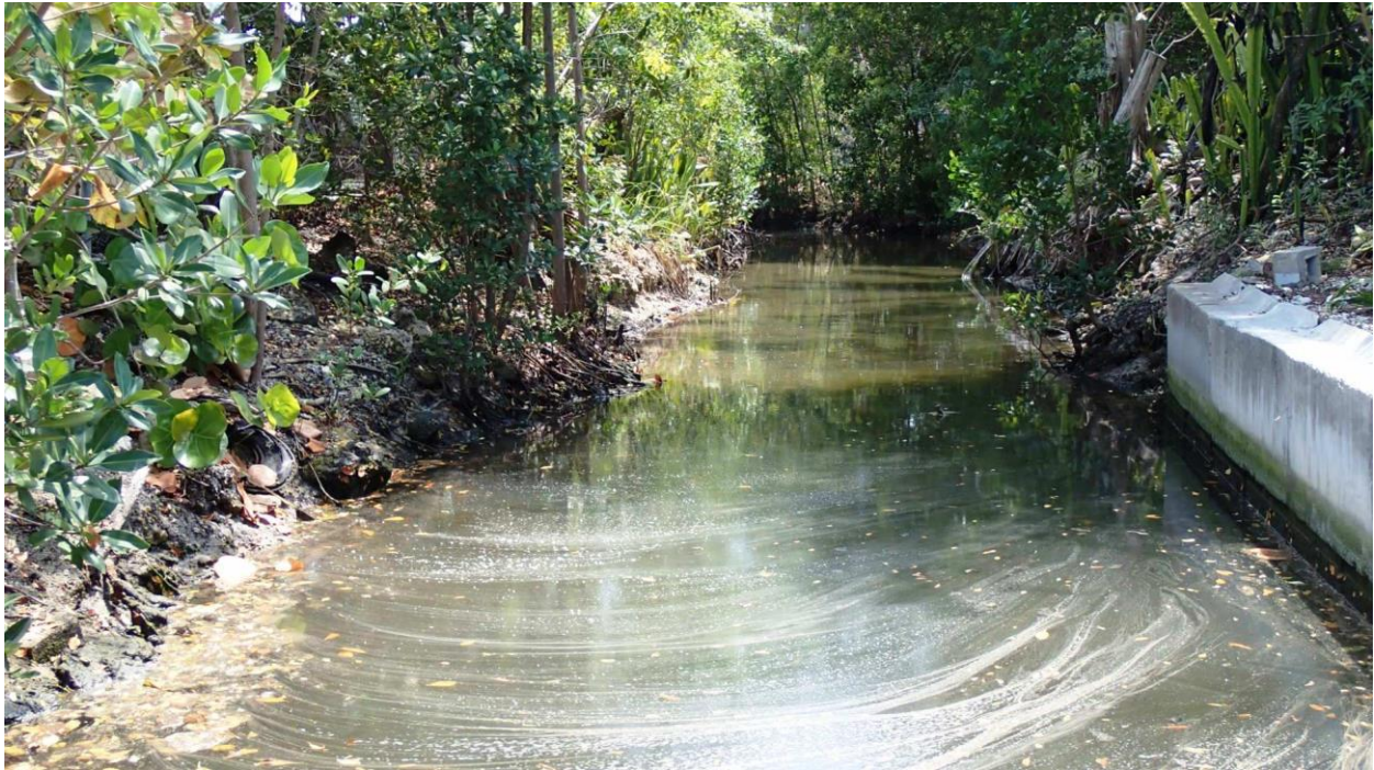
Photo of Linda Avenue showing surface accumulation and debris along the banks of the channel.
