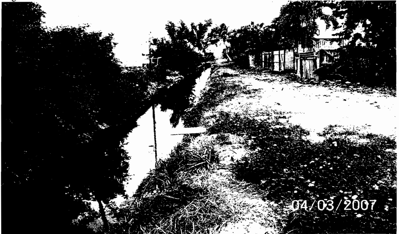
Photograph 6: Poinciana Donald Drainageway
