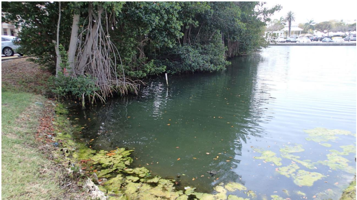
Photo of Jose Marti Pond showing scum accumulation and mangrove branches encroaching in pond.
