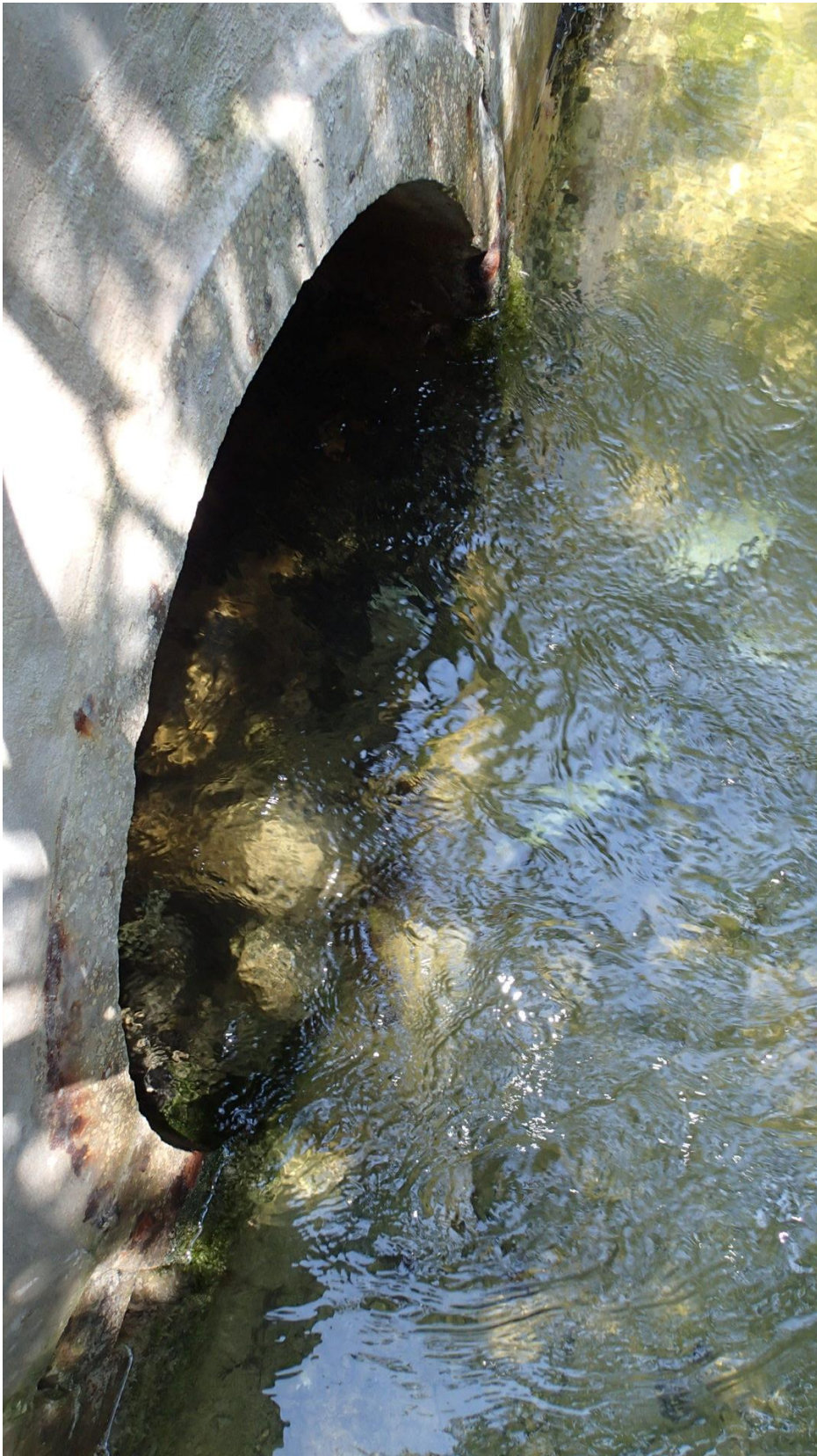
Photo of Government Road culvert showing culvert condition and optimal flow.
