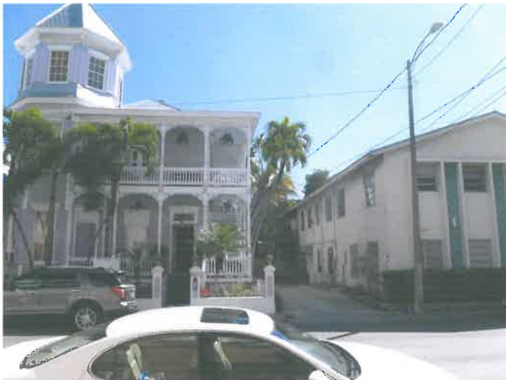
Adjacent Property (534 Eaton St.)
