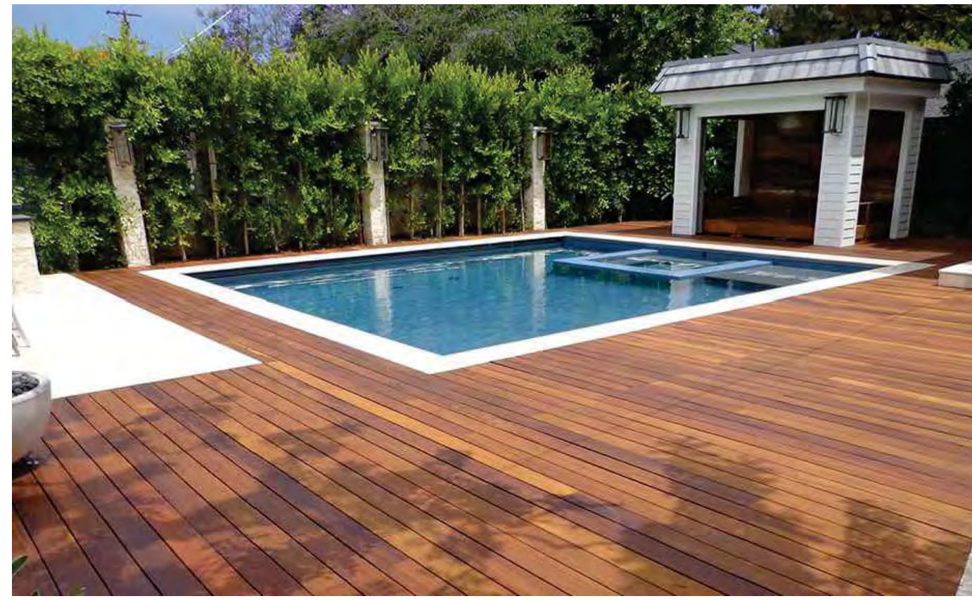
IPE POOL DECK WITH OILED FINISH AND CORAL-STONE SWIMMING POOL COPING
