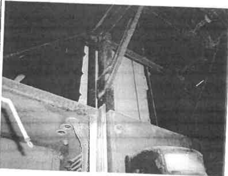
View of Transite panel in the switch station.
