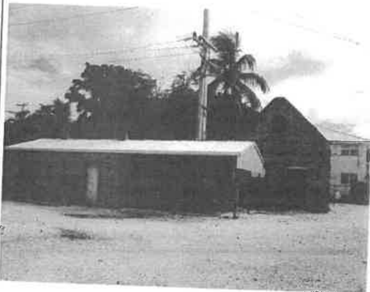
View of the Blacksmith Shop and Machine Shop
