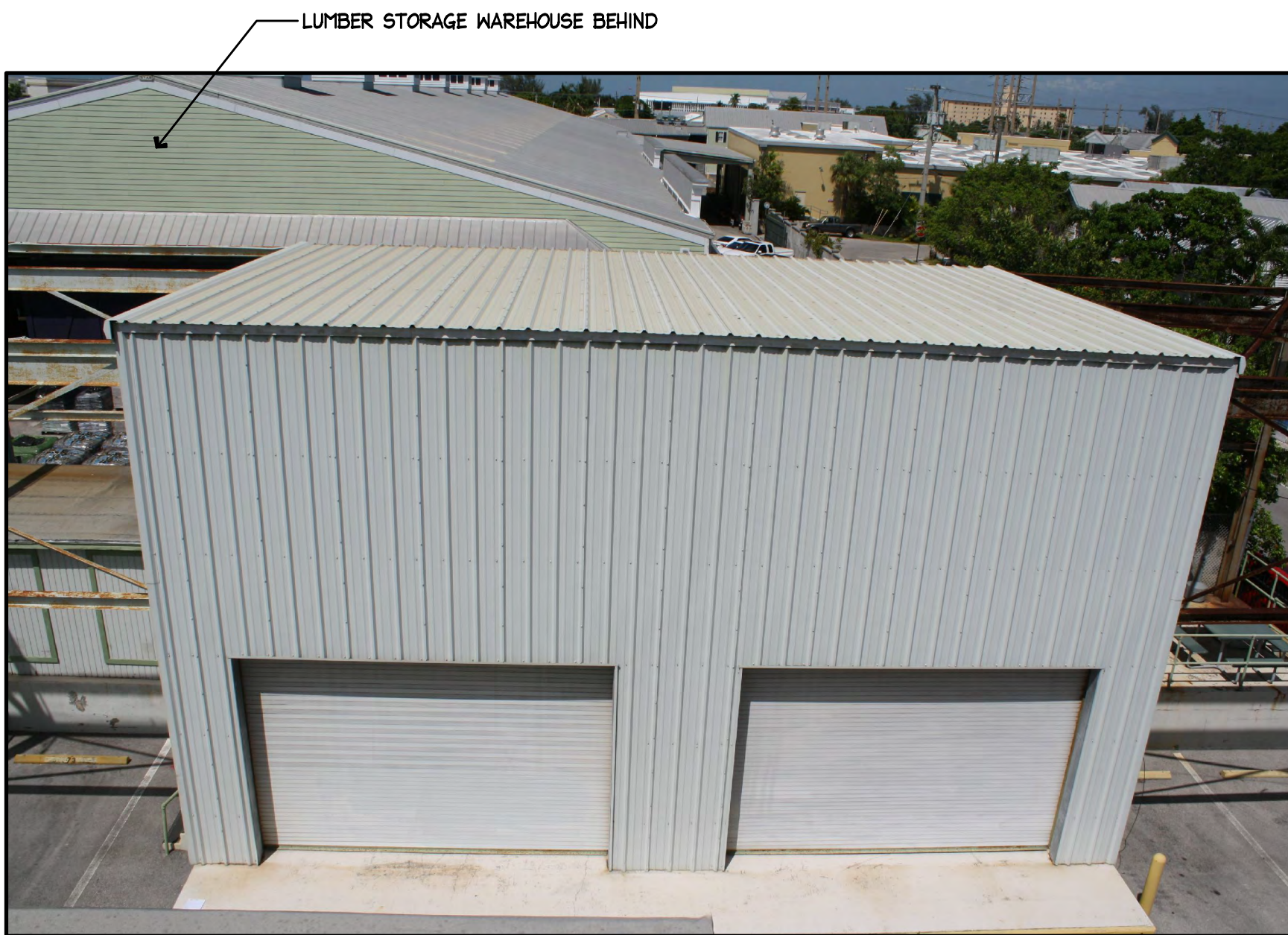
8 PHOTO OF EXISTING STRUCTURE A6.3 N.T.S.
