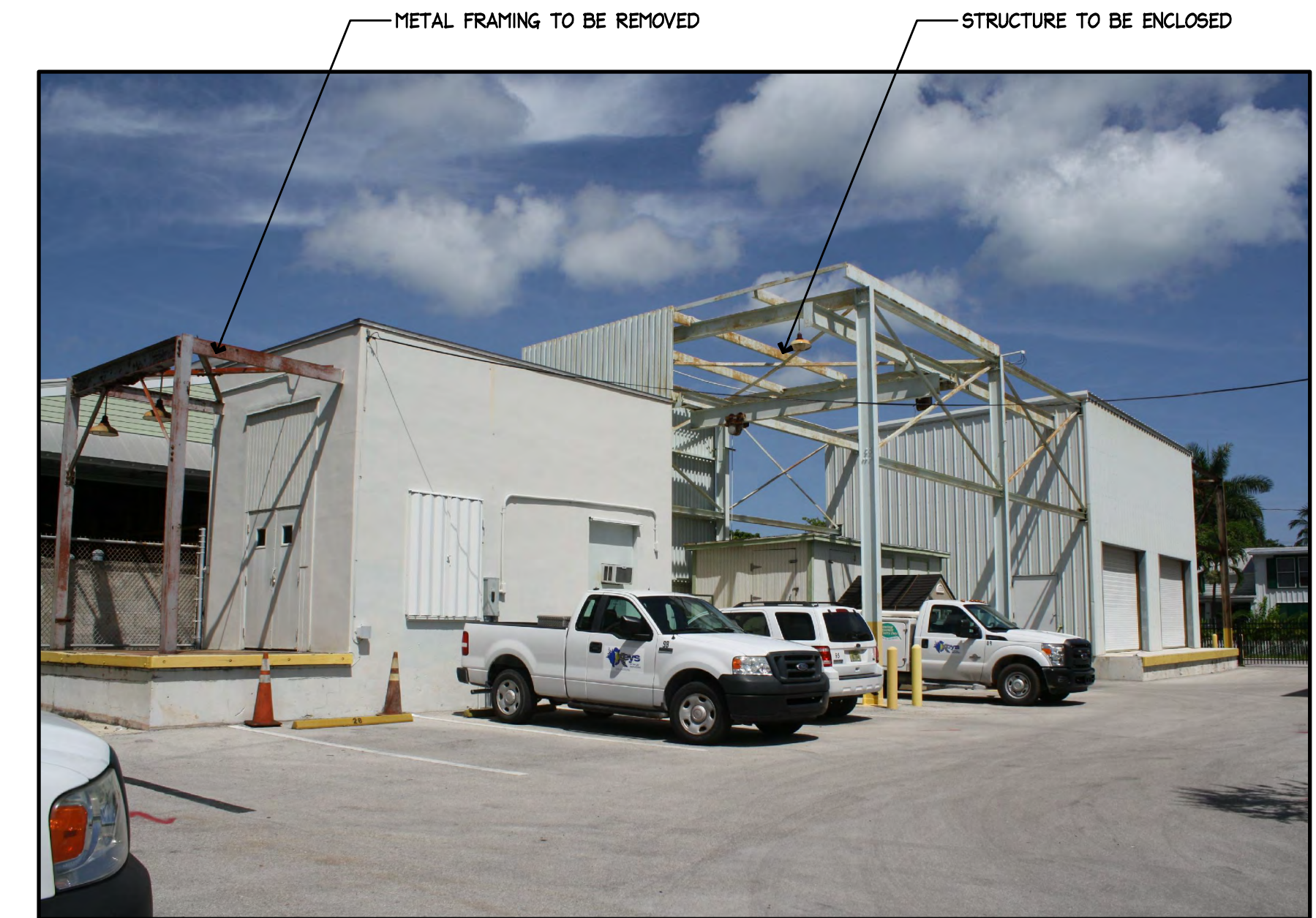
6 PHOTO OF EXISTING STRUCTURE A6.3 N.T.S.
