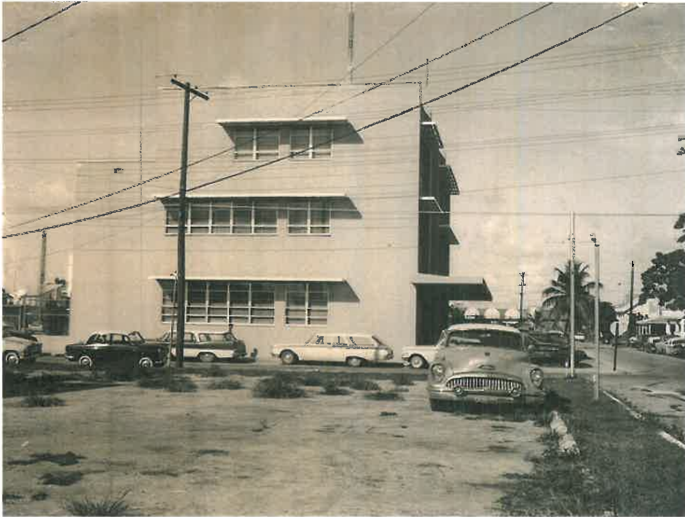
Photo taken by Property Appraiser's office c1965; 1001 James St.; City Electric System. Monroe County Library
