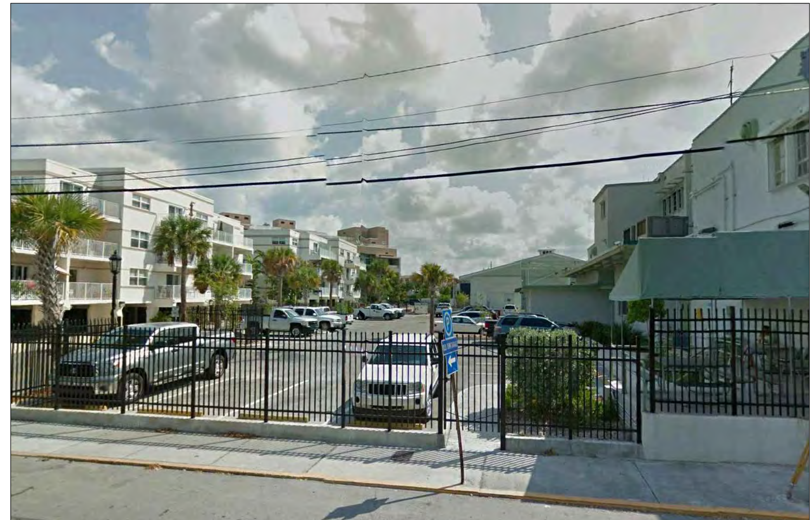
1 H3 KES PARKING LOT AND STEAMPLANT CONDOMINIUMS ADJACENT
