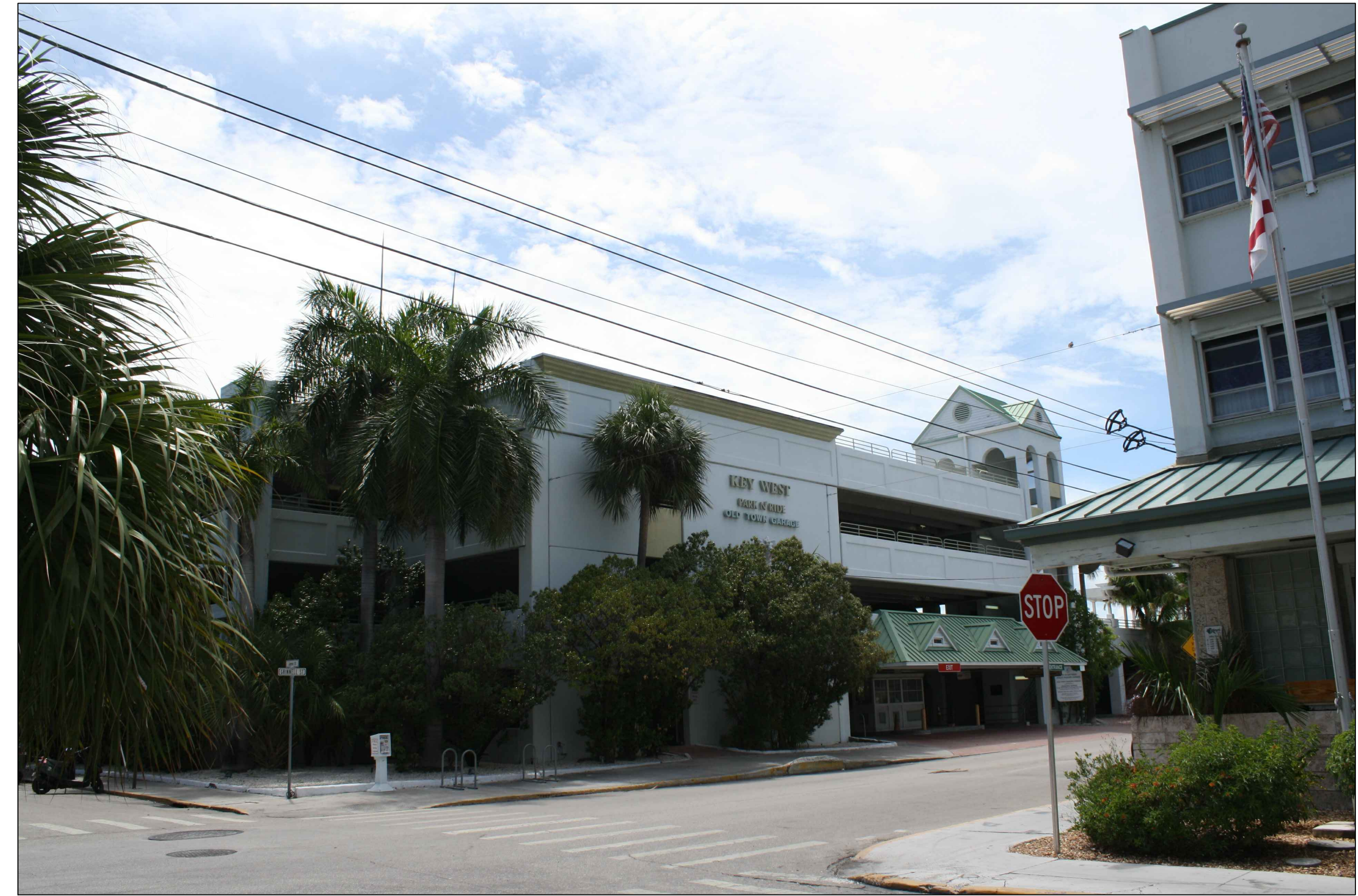
3 H3 PARKING GARAGE ACROSS JAMES STREET
