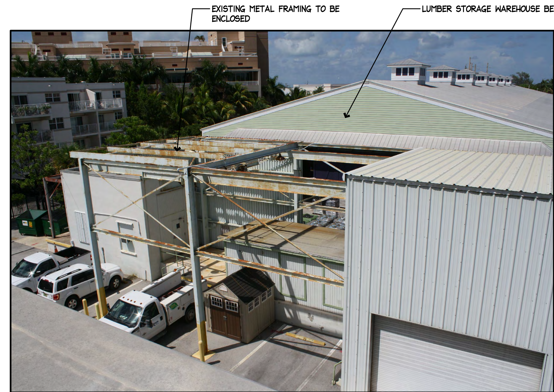
7 PHOTO OF EXISTING STRUCTURE A6.3 N.T.S.
