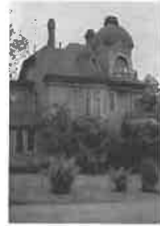
Special problems inherent in the design of an elaborate historic roof can be controlled through regular maintenance. The shape and detailing are essential elements of the building's historic character, and should not be modified, despite the use of alternative surface materials. Photo: NPS files.
