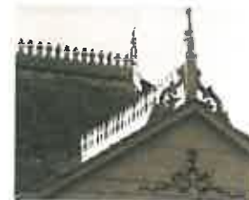
Decorative roofing feature. Photo: HABS Collection, NPS.
