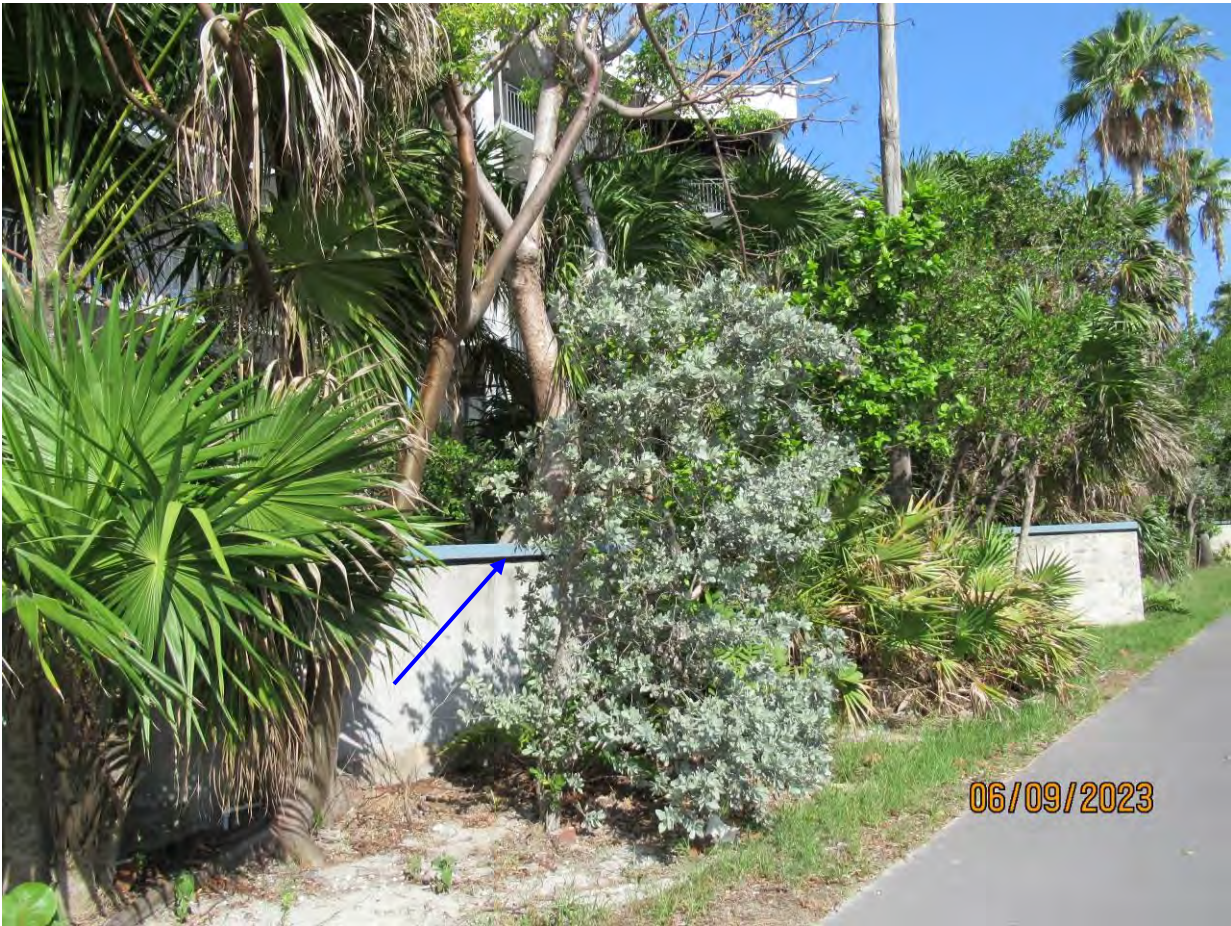
Photo showing location of tree trunk, view 1.
