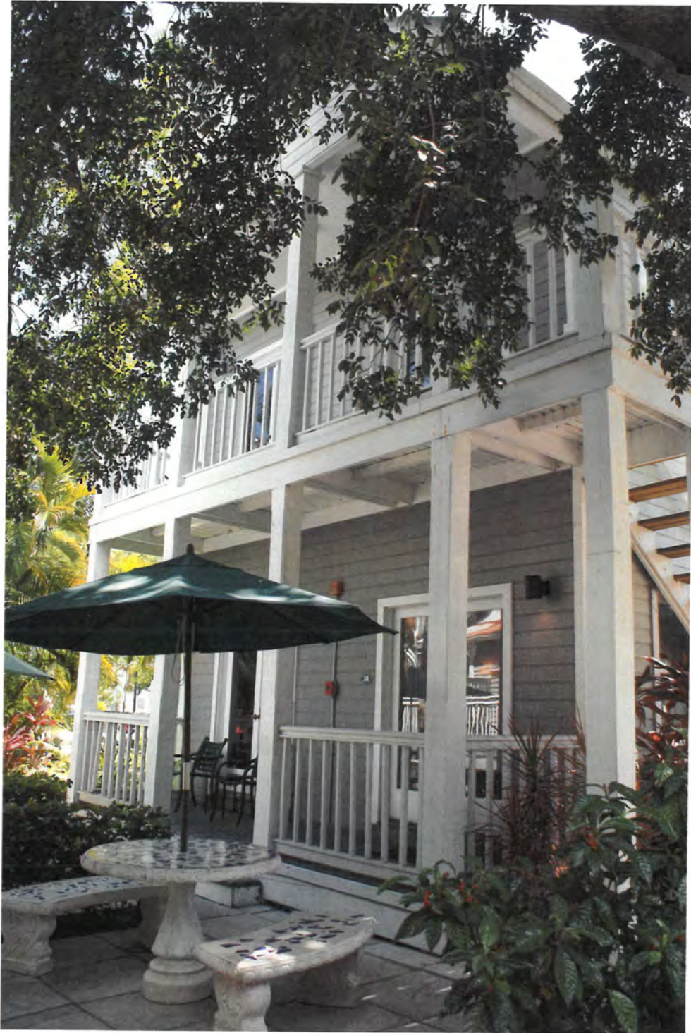
East - Before Construction (opposite Elizabeth Street)
