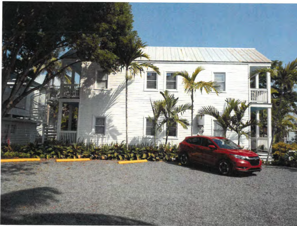
North - Rear View (opposite Truman Ave)
