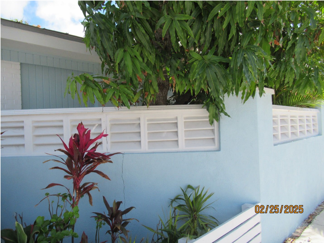
Photos of the crack on the concrete wall on the inside of the property and outside of the property
