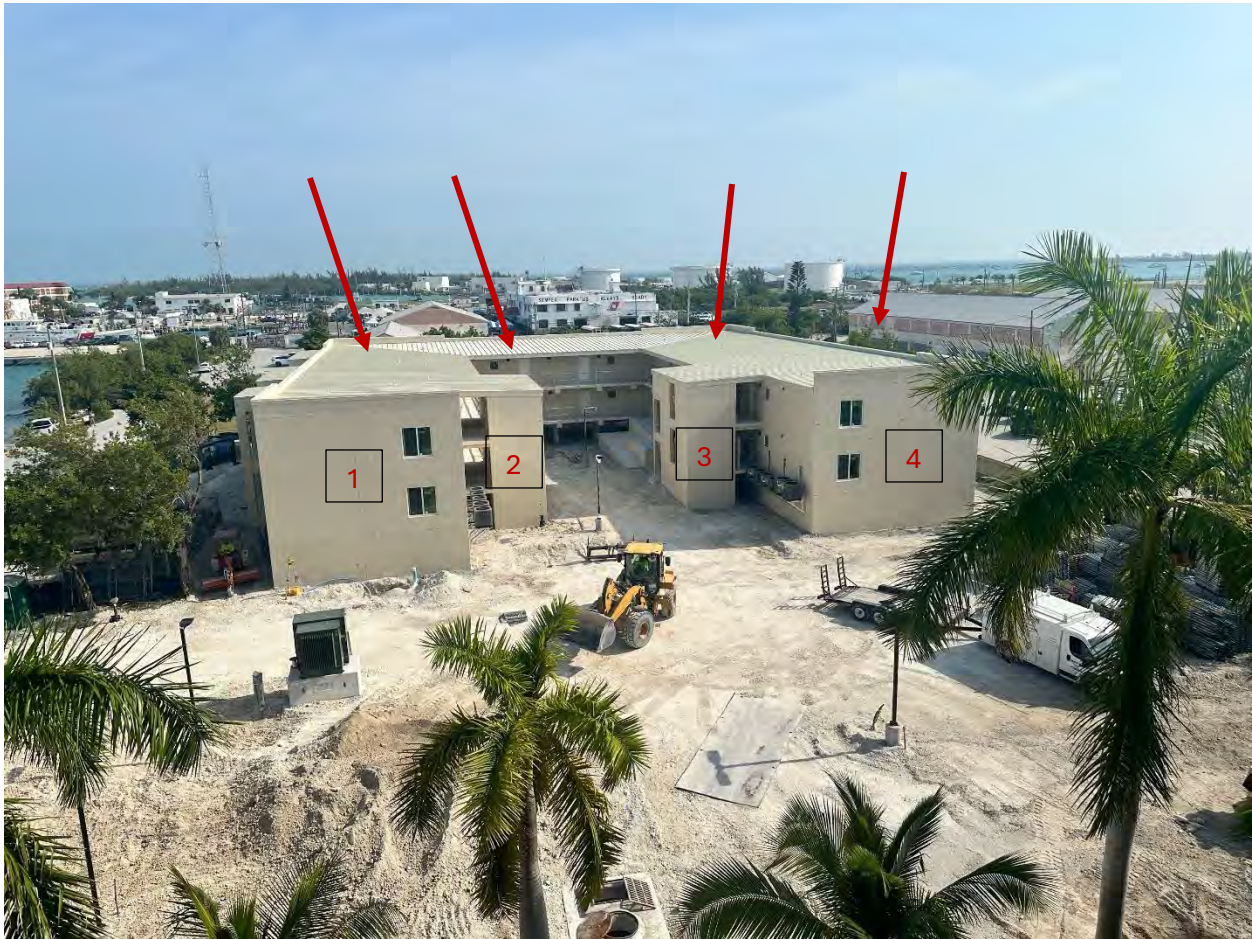
Walls under review.
