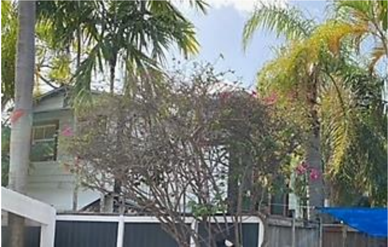
View looking at the front of 1011 Truman Avenue (rear) where the proposed work will occur.
