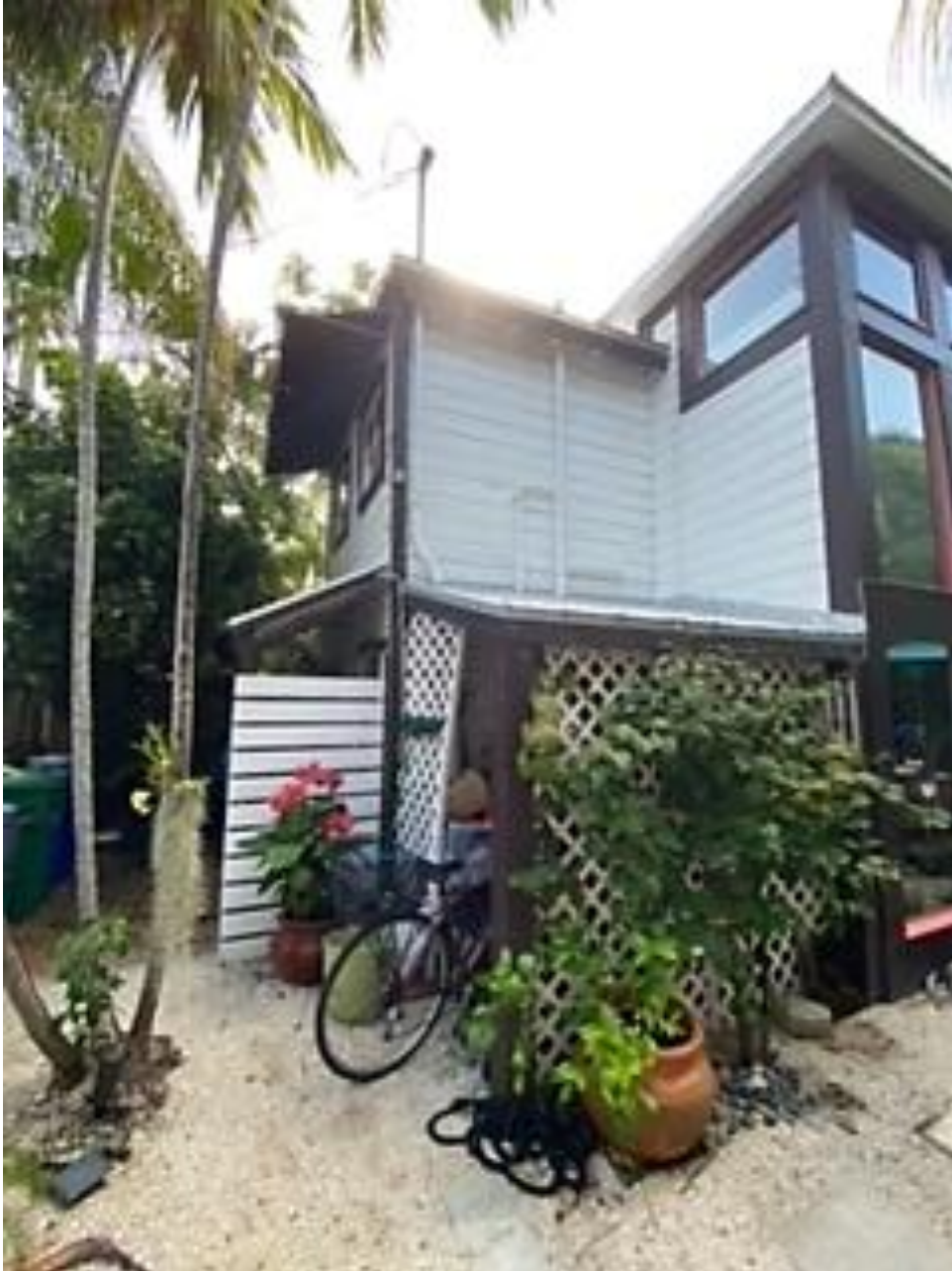
View of the side of the 1011 Truman Avenue (rear) structure where the work will occur. Two shed roofs are shown.
