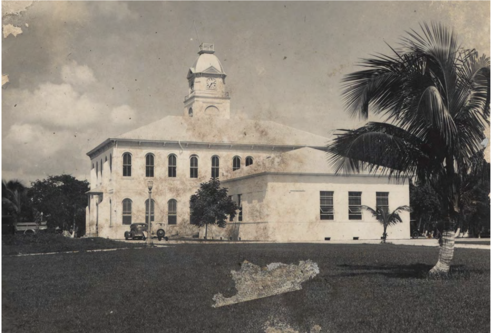
Rear of Monroe County Court House circa 1940. Monroe County Library.
