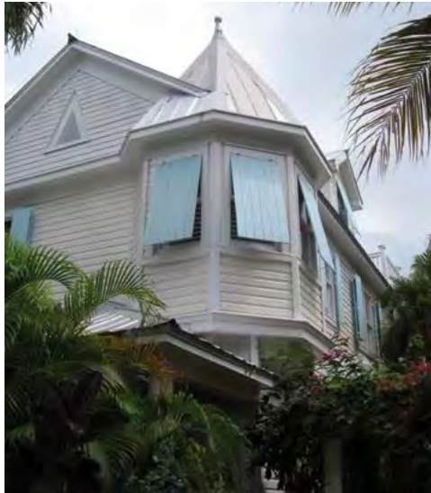
[30] Historic window shutters still serve their original function as protection in hurricane-prone areas.
