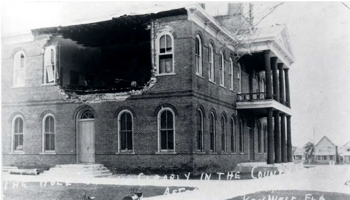
Monroe County Courthouse after 1919 hurricane. Monroe County Library.
