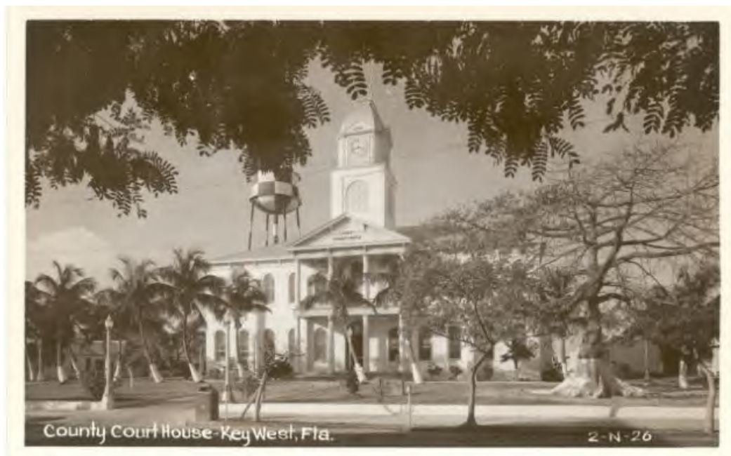
1940's photo of courthouse. The building was painted white in the 1940s. The paint was then sandblasted off in the 1950's, severely damaging the bricks.
