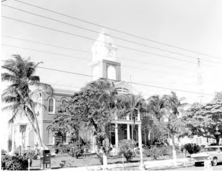
Circa 1960 photo of the building. Paint has been removed.
