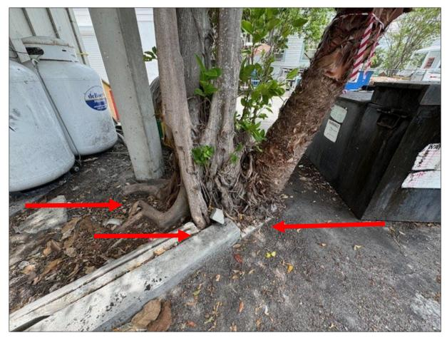
Roots are exploding from the cement cub and into the parking lot and toward the structure and tanks.
