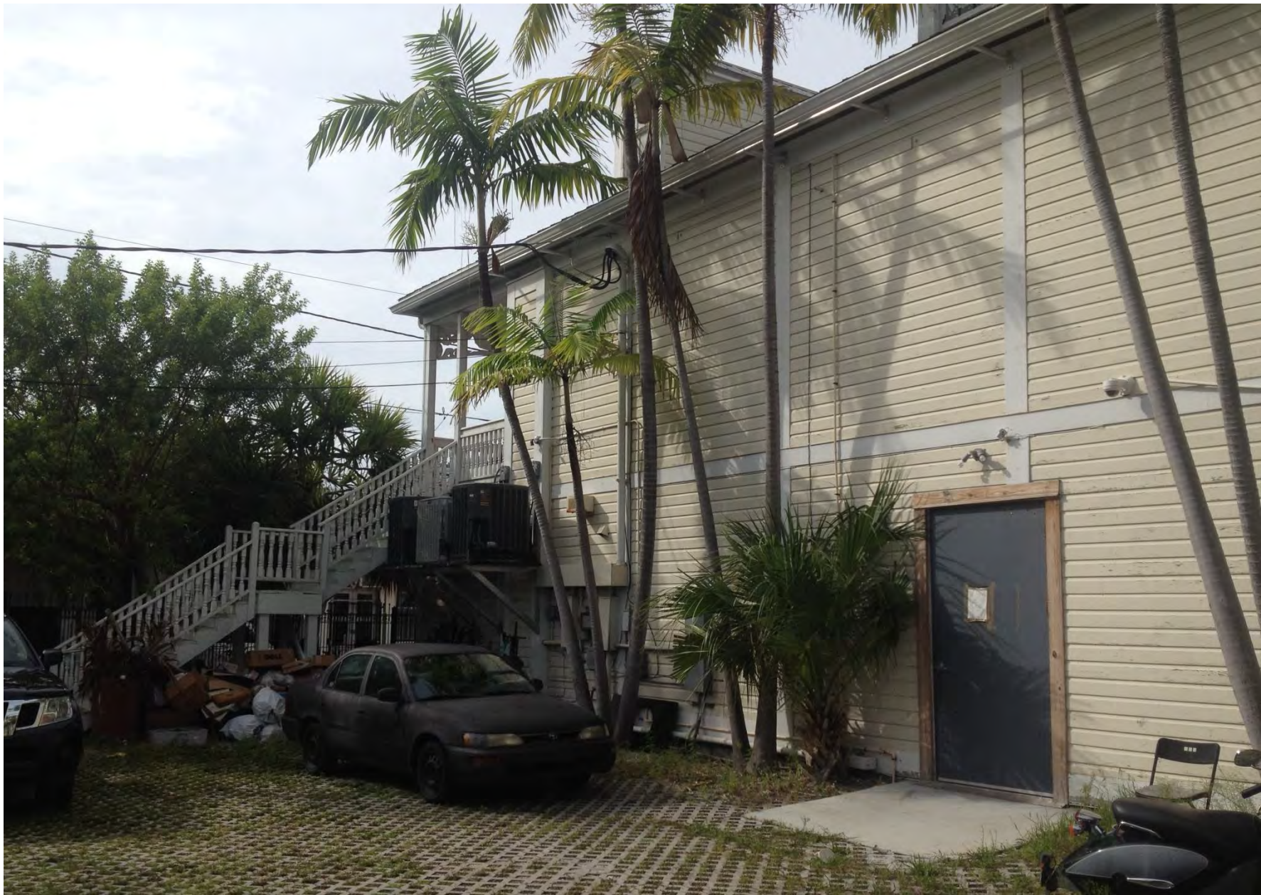
725 Duval Street PARTIAL REAR VIEW
