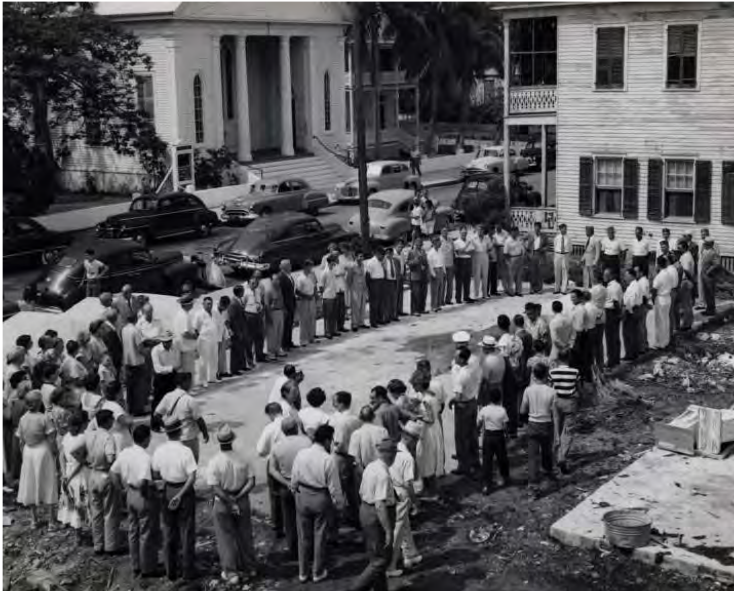
Ground breaking for the Scottish Rite Masonic Temple July 1950. Monroe County Library
