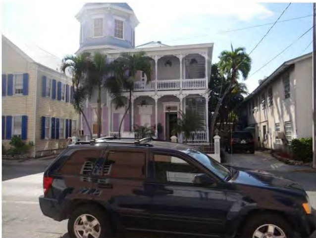
View across Eaton Street looking South toward Artist's House
