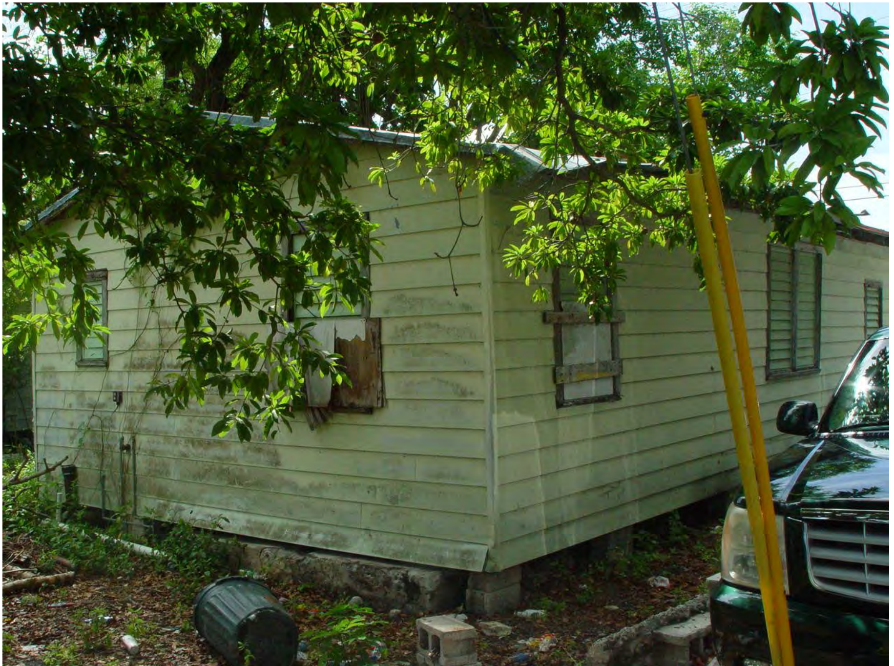
Photograph from 2008 showing structure before it was demolished.
