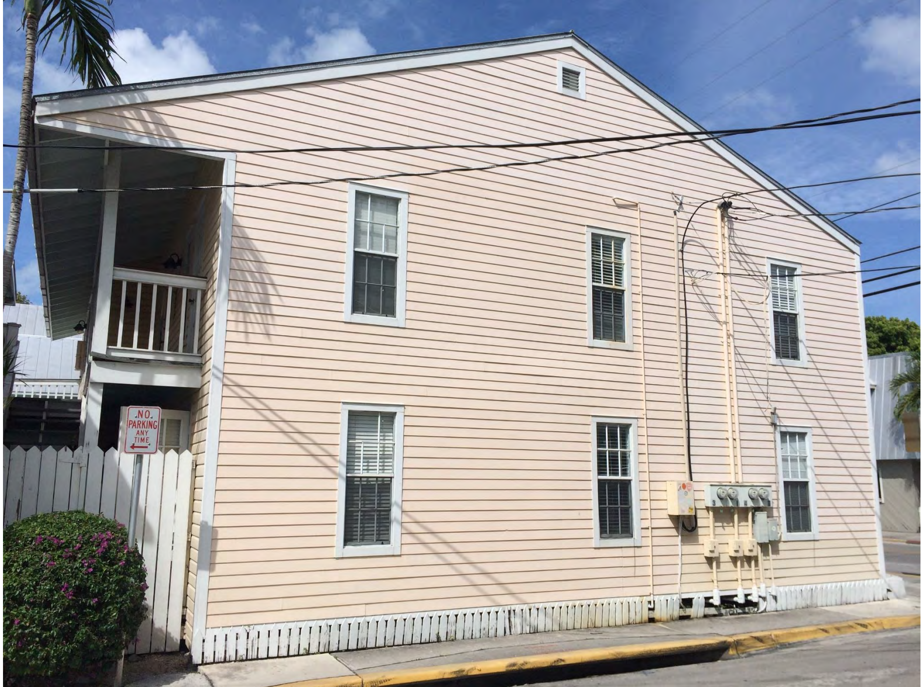
632 Whitehead located at the corner of Angela Street and Whitehead Street
