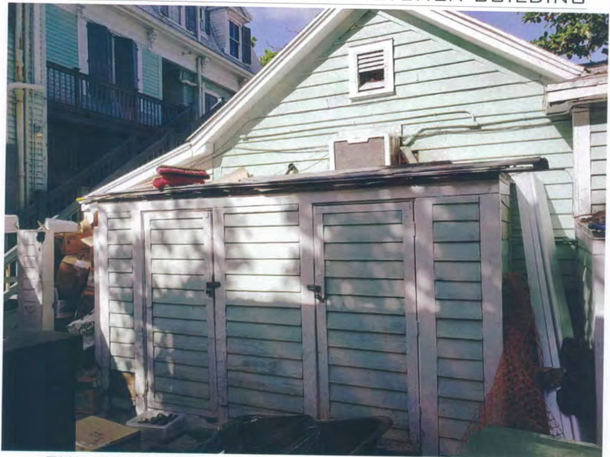
EXISTING CONDITIONS REAR VIEW OF PROPOSED KITCHEN BUILDING
