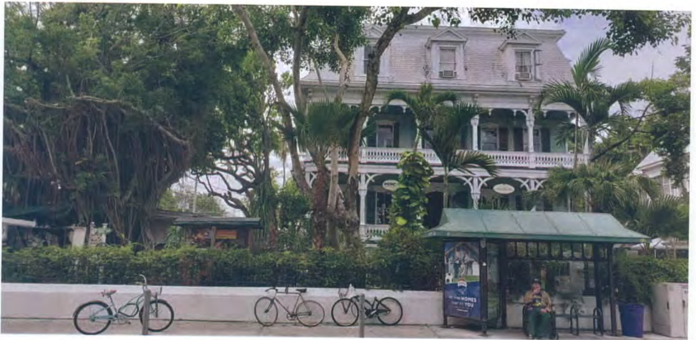
EXISTING CONDITIONS OVERALL VIEW FROM CAROLINE ST
