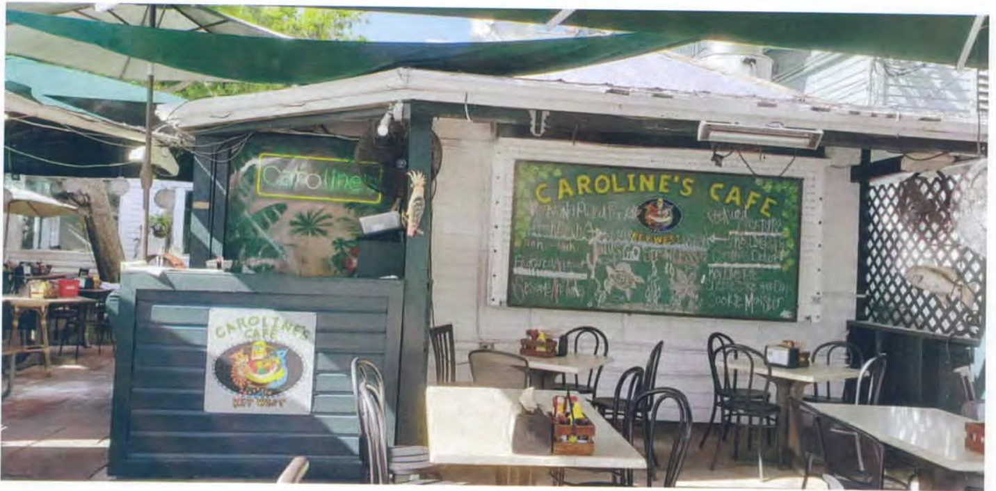
EXISTING CONDITIONS FRONT VIEW OF PROPOSED DINING PAVILION (FROM DUVAL ST)
